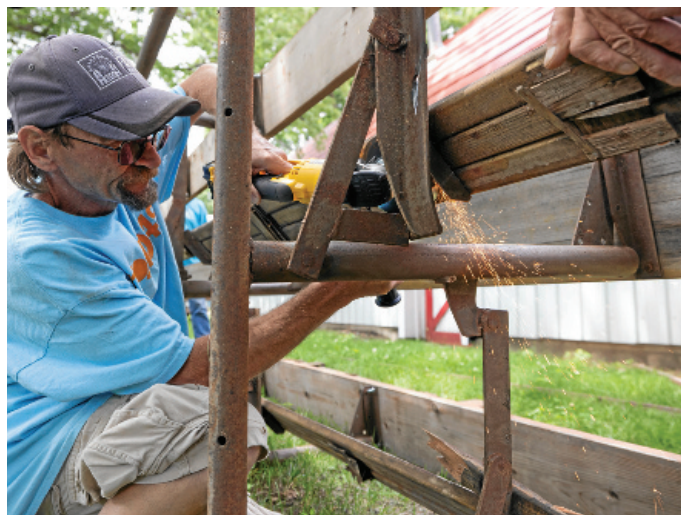
Dan Alspach cuts off rusty bolts in order to install new boards and modernize these bleachers before the Clay County Fair opens.
