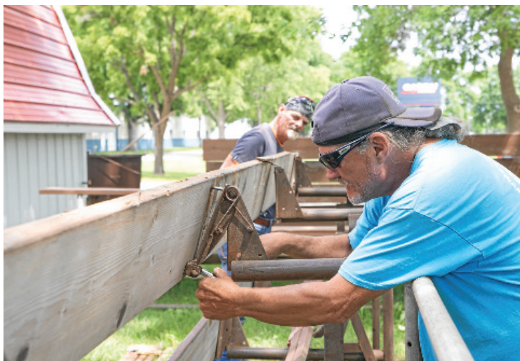
Randy Johnson removes the old bolts on these bleachers to install new boards as they prepare for the Clay County Fair in Spencer, Iowa.
