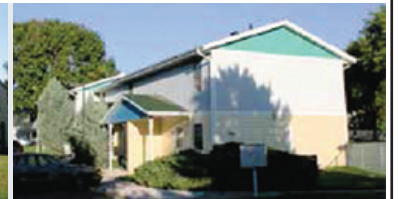
TOWNVIEW APTS (32 units) 2 and 3 BR Apts 400 West 4th St. • Sioux City, IA. 51103
