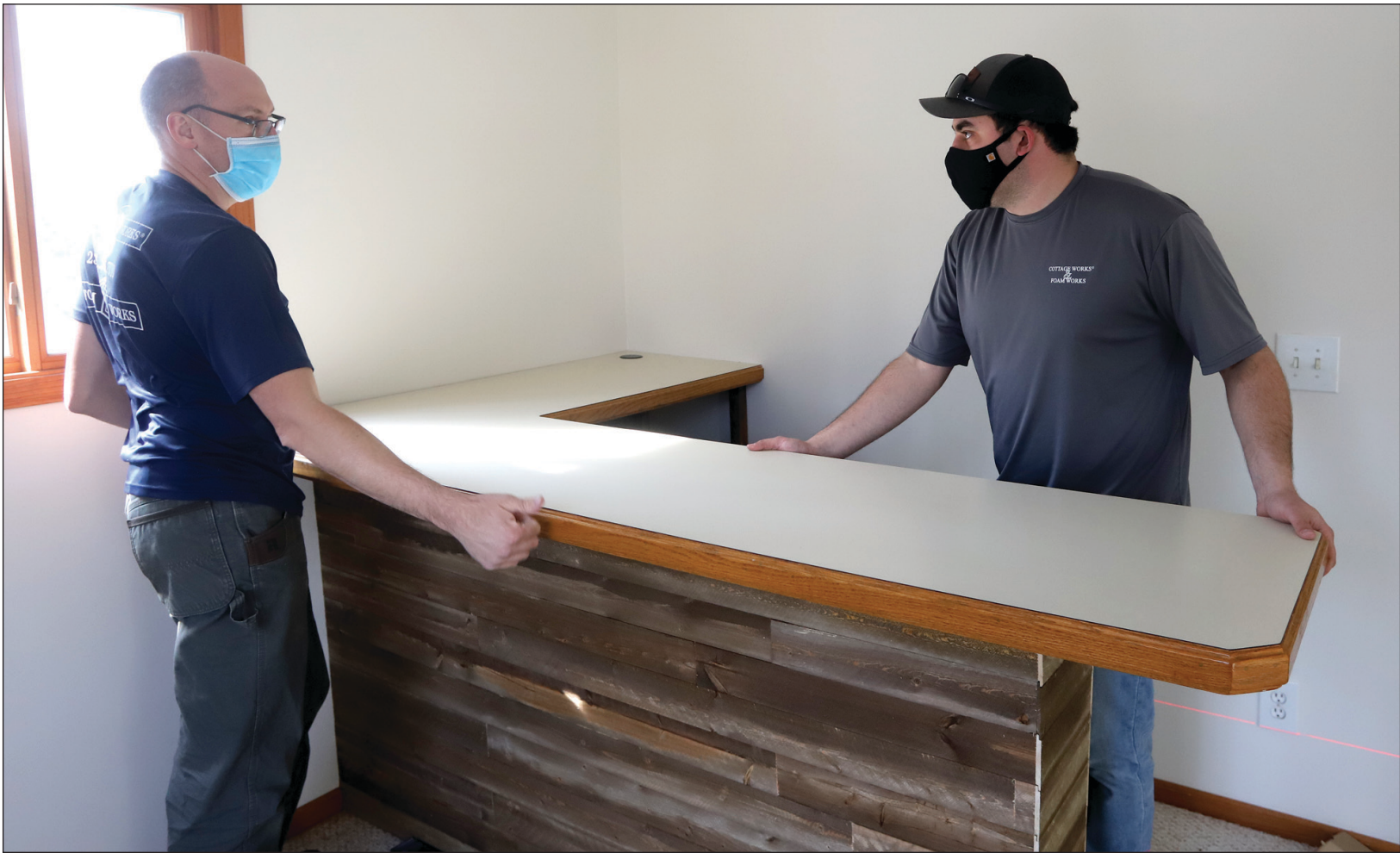
Chris Dudle and Jon Wittlieff, employees at Cottage Works, move the bar top into place and attach it during the room redo.
