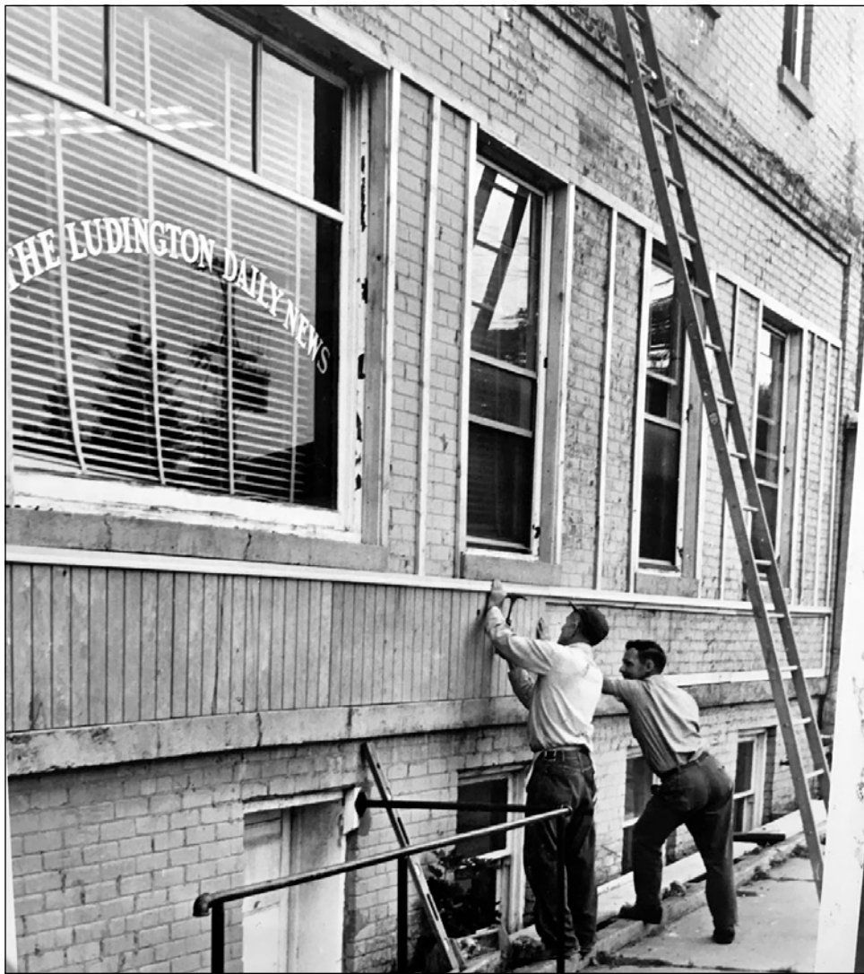
Workers make repairs to the Ludington Daily News offices, located at the intersection of Rath Avenue and Court Street.
