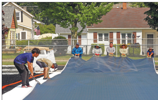
Workers pull a portion of the artificial turf into place at Oriole Field in early August.
