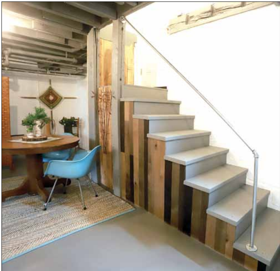
The stairs leading down to the basement were done to provide a stable entry into the gathering space. The team encased the stairs with ship lap and cedar, and added a hand rail. They painted the treads, adding a non-slip tape.
