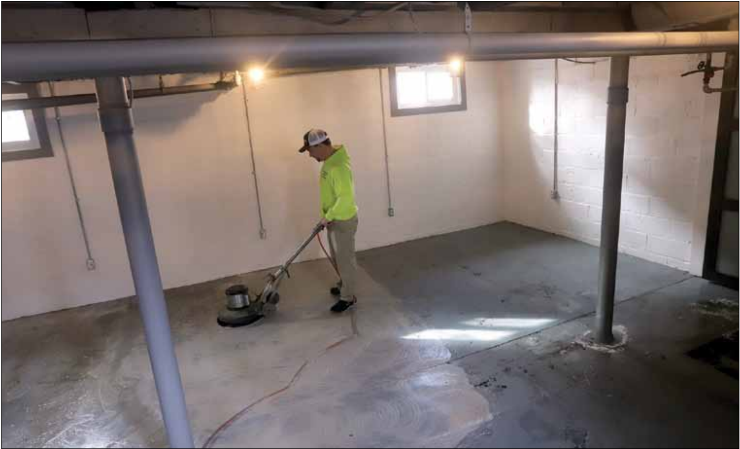
Jason Muralt of ProMaster scrubs the basement floor before it was painted. The basement floor had some areas of grease and dirt that needed to be cleaned before Van Dyke could put down the final coat of paint.
