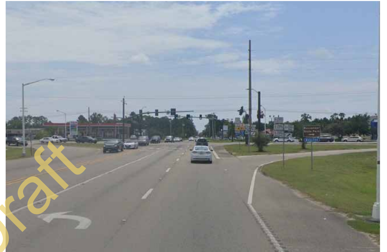
Welcome and wayfinding signs overwhelmed by the large scale of the intersection
