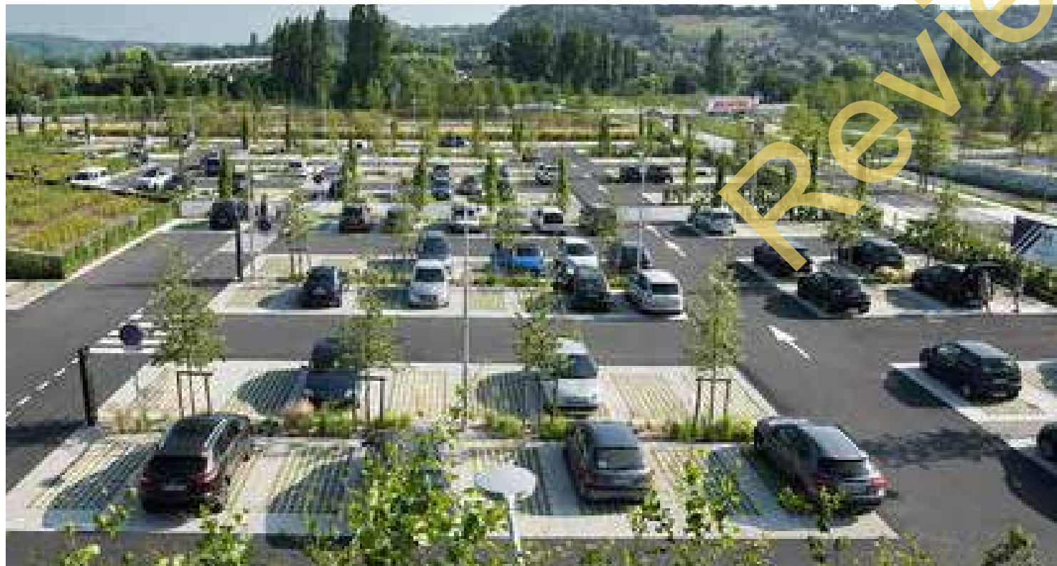
Parking lot retrofit
