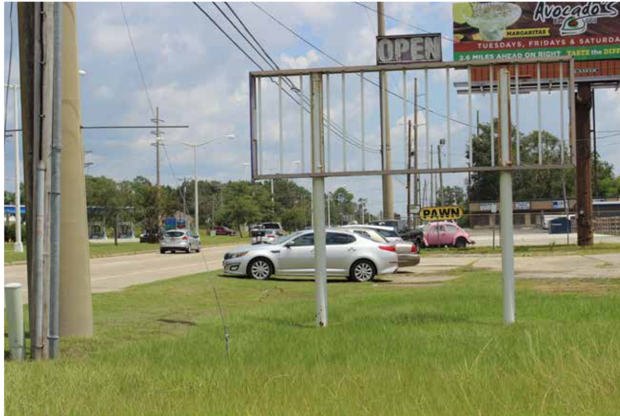
One of nearly 50 abandoned signs in the corridor
