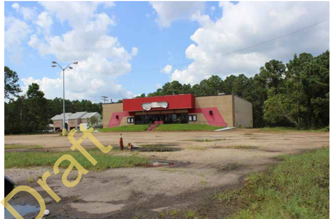
Abandoned signage on a vacant building
