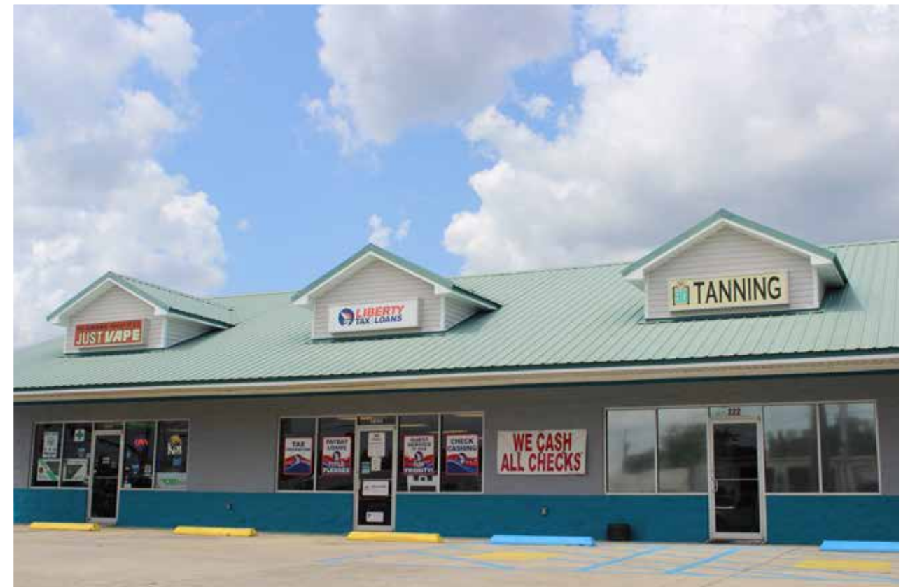
Temporary banners create a visually cluttered corridor
