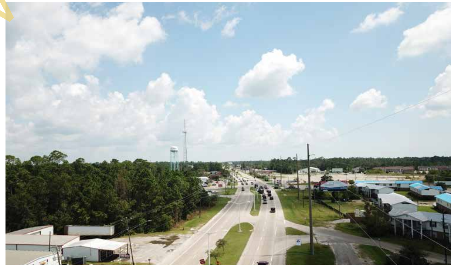
Corridor looking west
