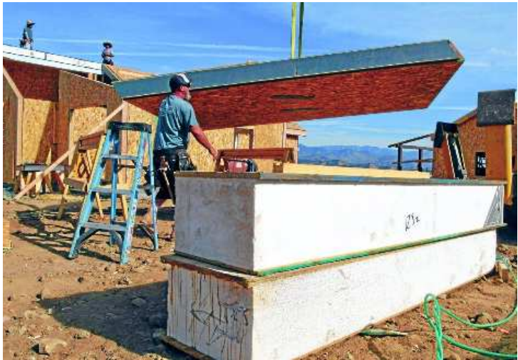
LEN WOOD, STAFF Two SIP post panels made of a sandwich of structural board and rigid foam are stacked as a larger roof panel is lifted onto a staff residence under construction at Rancho Alegre Boy Scout Camp. The popular Outdoor School and Scouting facility is rebuilding after virtually total destruction from the Whittier fire in July 2017.
