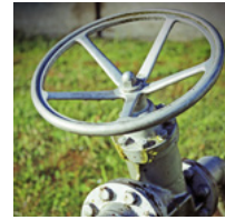
ELIMINATE METHANE GAS LEAKS
