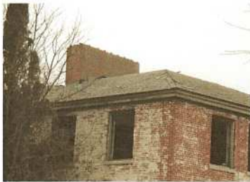
Roof East and Northeast
