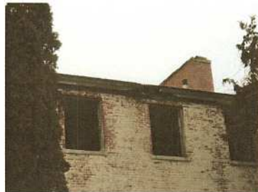
Roof Trim and Chimney Northeast
