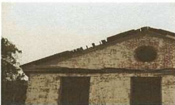
Front Roof South Side
