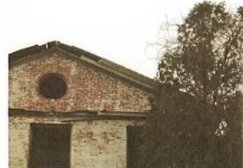
Front Roof North Side
