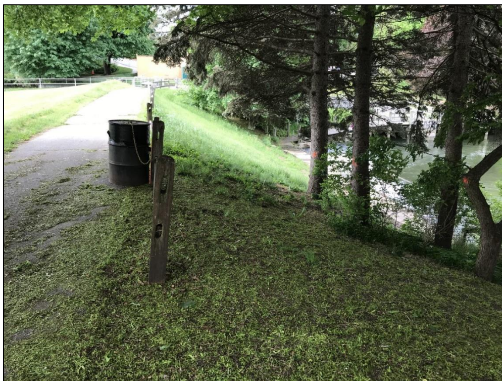
Photograph 35 – Downstream slope from right abutment. Note trees.
