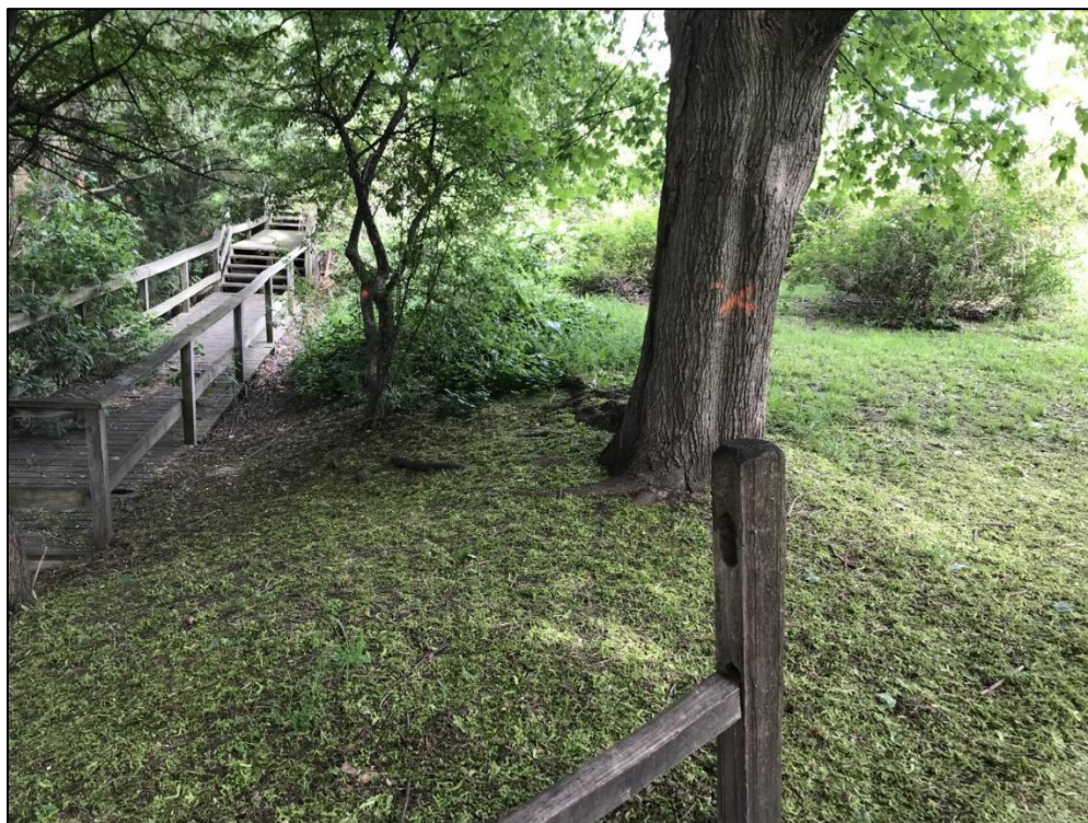
Photograph 36 – Looking at right abutment and downstream bank from crest.
