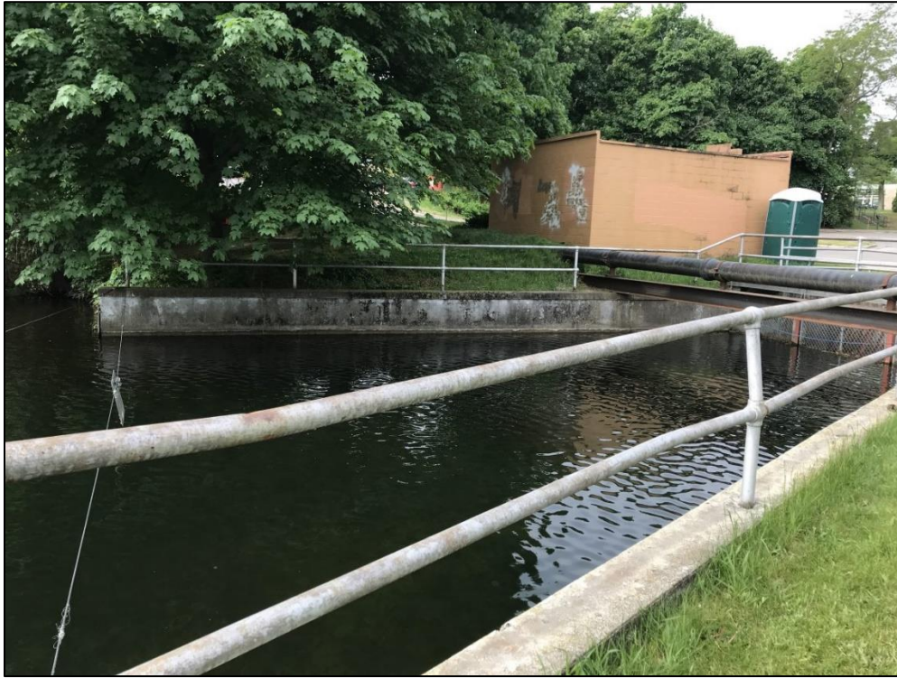
Photograph 21 – Left auxiliary spillway wingwall viewed from right wingwall.
