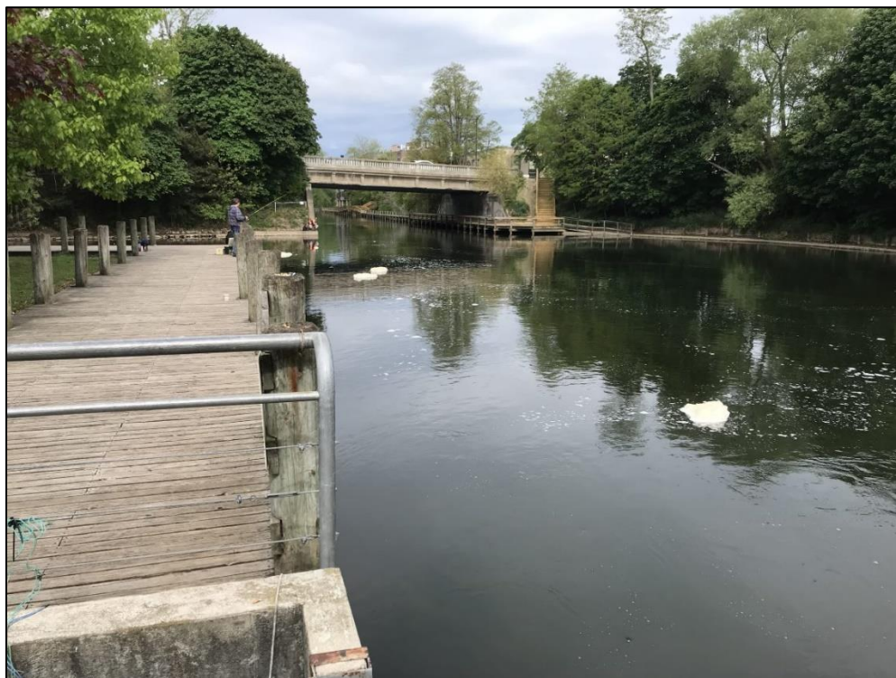
Photograph 53 – Left bank of downstream river channel with boardwalk.
