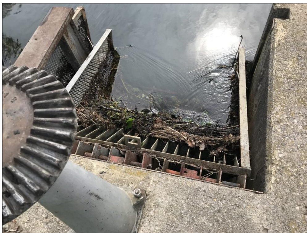
Photograph 27 – Left center bay of primary spillway intake.
