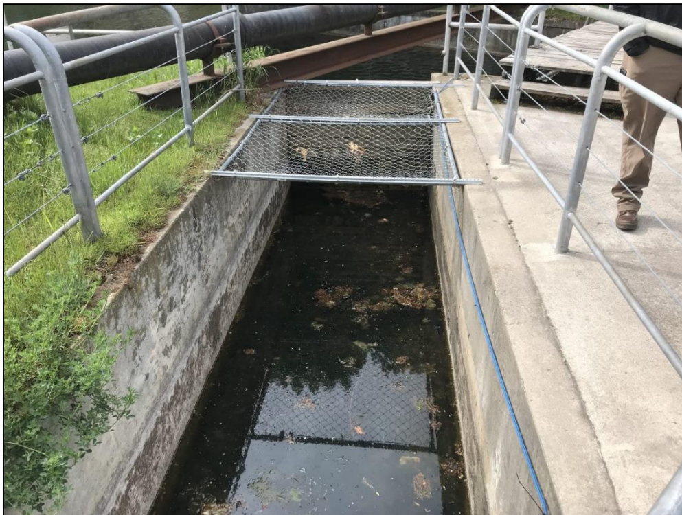
Photograph 12 – Looking at upstream fish ladder entrance from pedestrian bridge.
