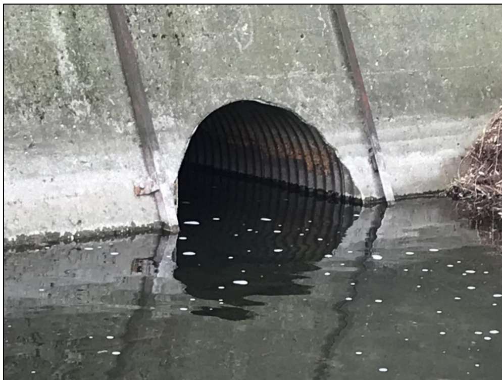
Photograph 57 – Left auxiliary spillway culvert outlet.
