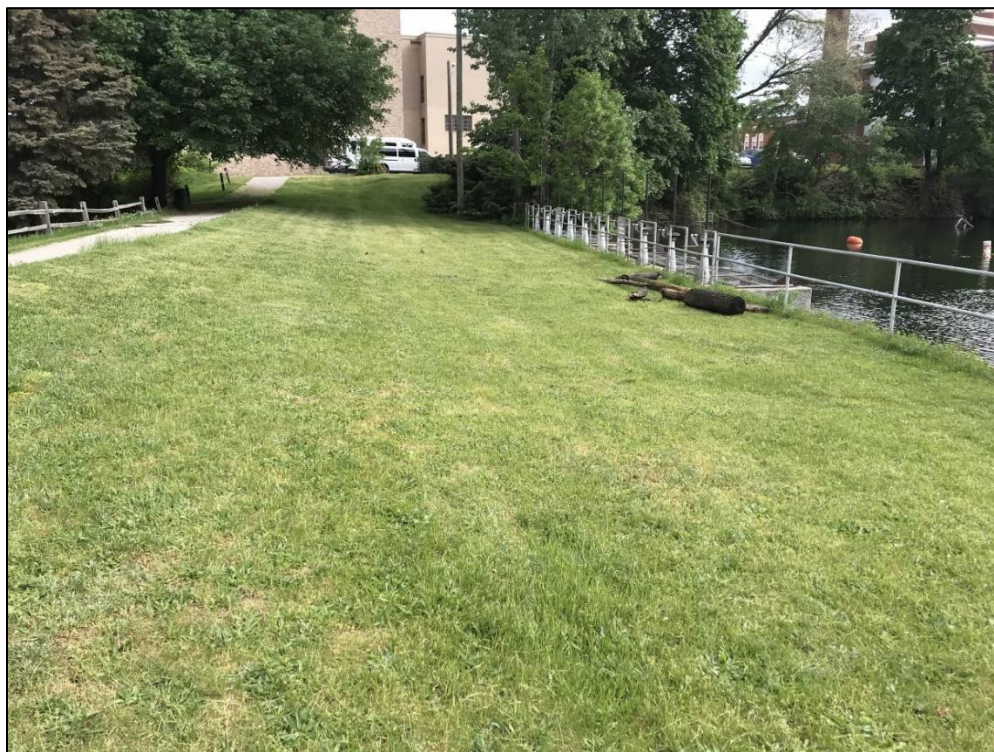
Photograph 17 – Downstream slope of embankment viewed from fish ladder.
