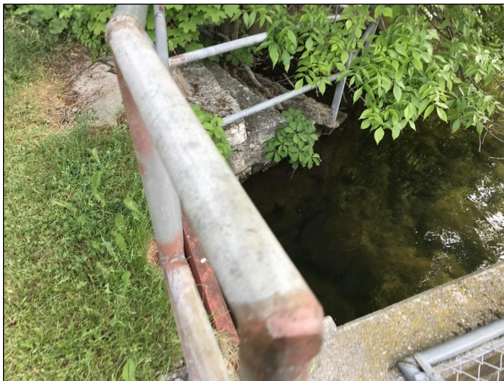
Photograph 30 – Upstream right abutment. Note submerged steps and walkway.
