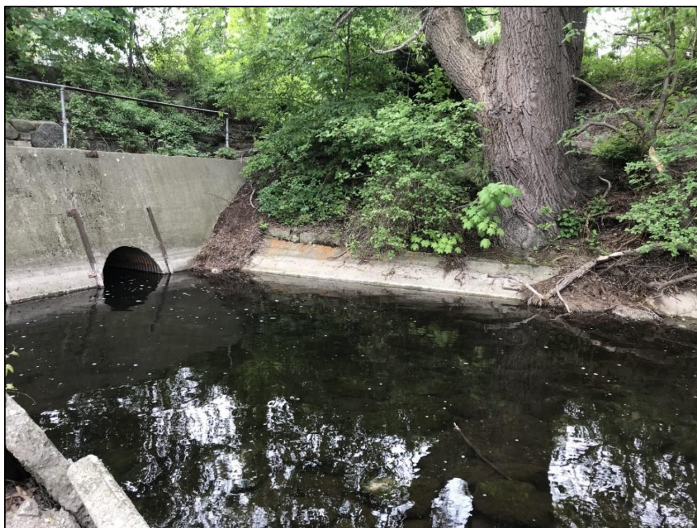
Photograph 56 – Left bank/wingwall of auxiliary spillway outlet.
