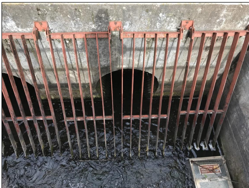
Photograph 8 – Right auxiliary spillway culvert inlet.
