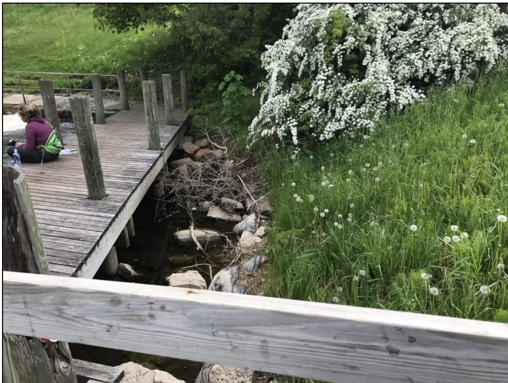
Photograph 46 – Toe of embankment between primary spillway and fish ladder.
