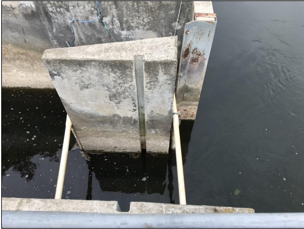
Photograph 49 – Downstream entrance to fish ladder.
