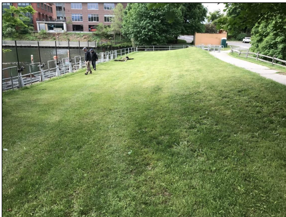
Photograph 33 – Upstream slope viewed from right abutment.
