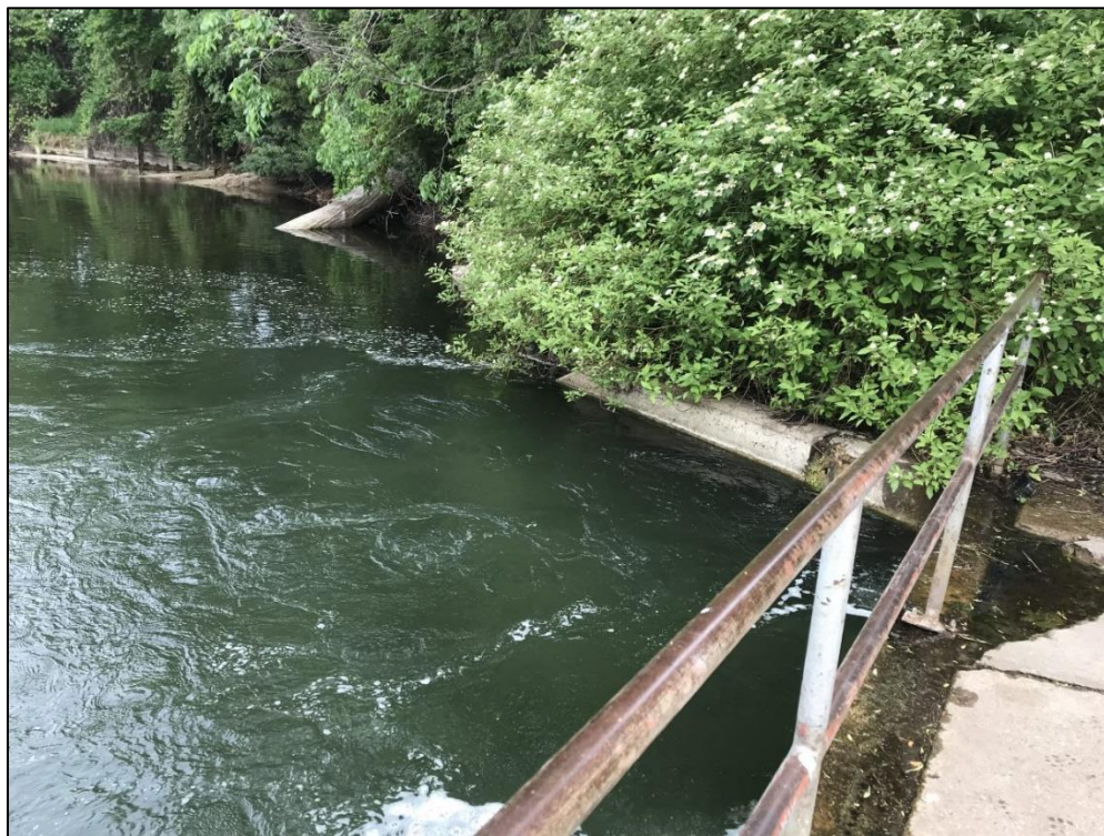
Photograph 41 – Downstream right bank. Note extensive vegetation.
