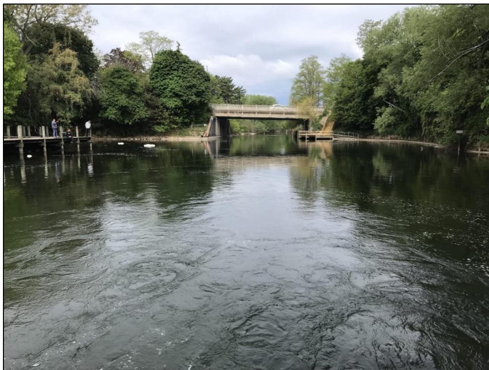
Photograph 40 – River channel downstream of primary spillway.
