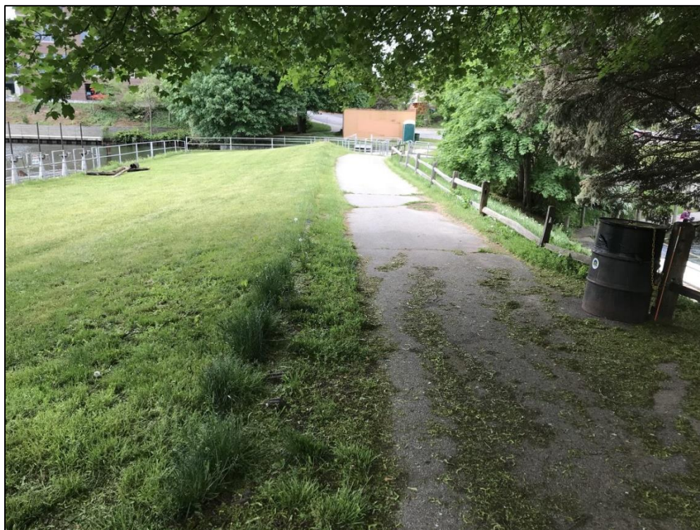
Photograph 34 – Crest viewed from right abutment.
