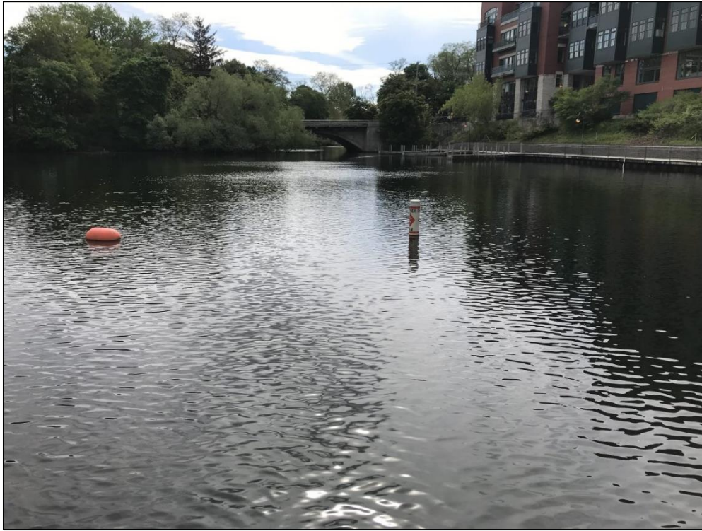
Photograph 19 – Impoundment upstream of dam.
