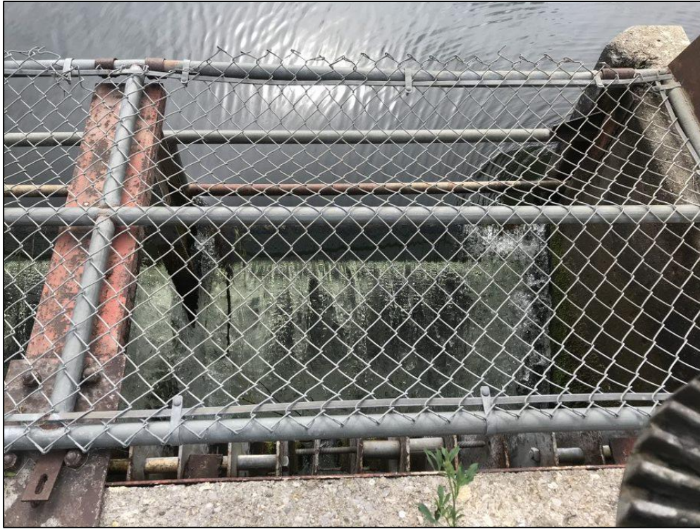
Photograph 24 – Looking upstream at left most bay of primary spillway intake.
