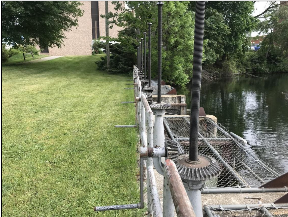
Photograph 25 – Upstream face of embankment and primary spillway.
