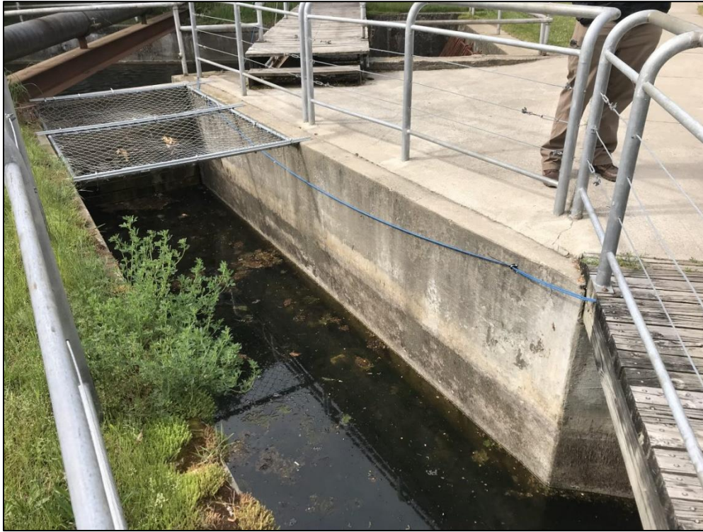
Photograph 13 – Left wall of fish ladder, looking upstream.
