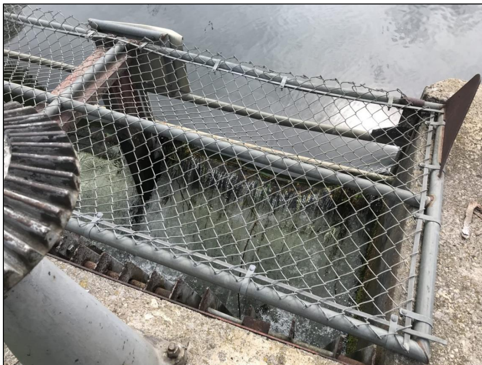
Photograph 26 – Looking upstream at third bay from left of primary spillway intake.
