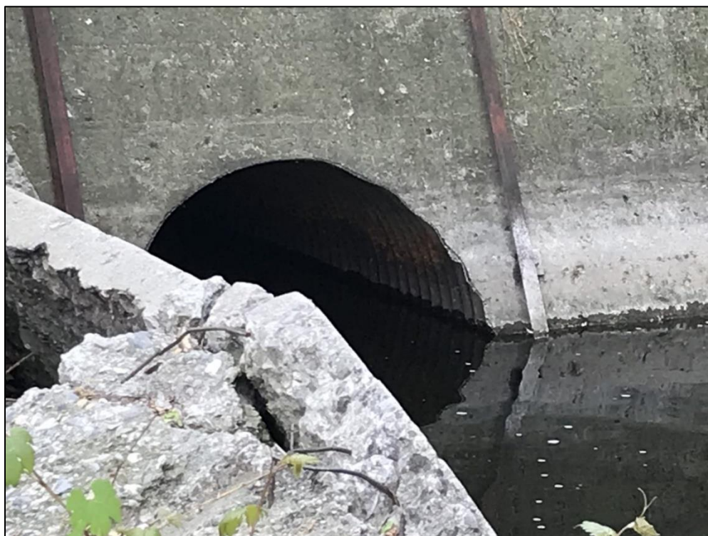
Photograph 58 – Right auxiliary spillway culvert outlet
