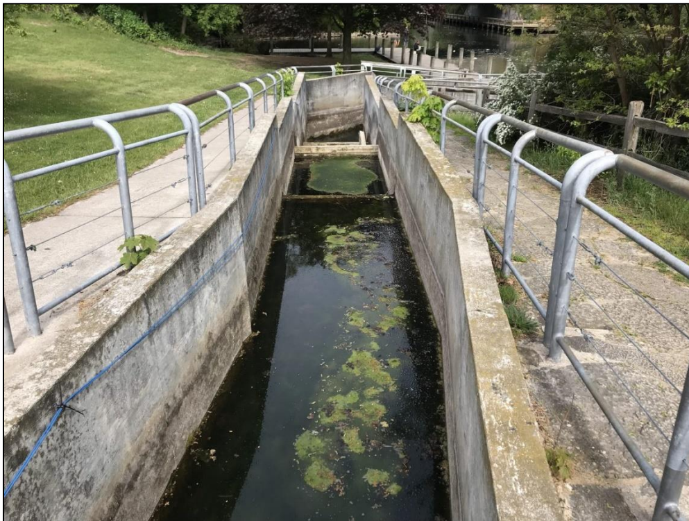
Photograph 14 – Looking downstream fish ladder from pedestrian bridge.
