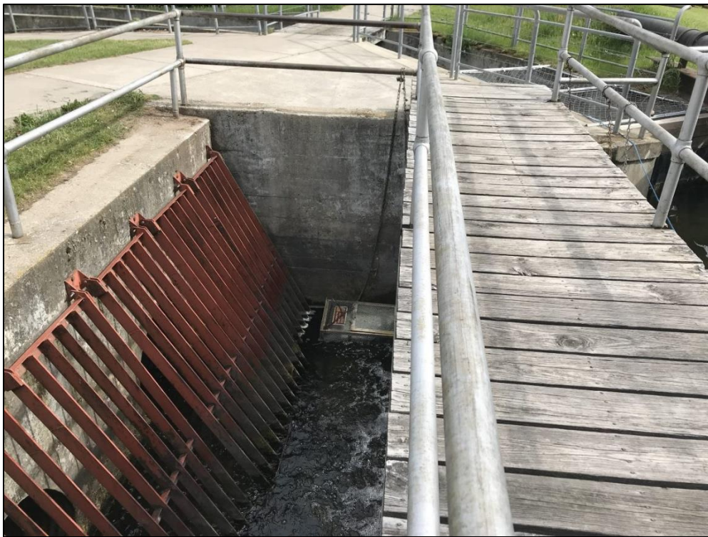
Photograph 6 – Inlet to auxiliary spillway culverts with trash racks.
