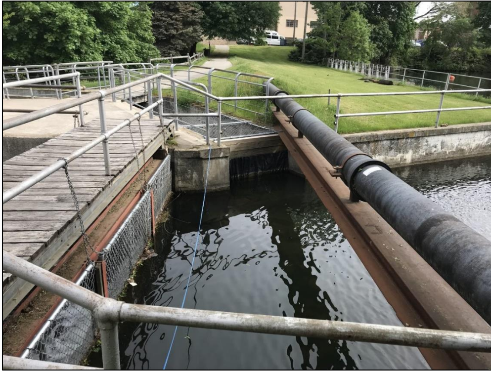
Photograph 5 – Upstream face of auxiliary spillway and fish ladder. Note fencing on spillway and fish ladder to prevent fish passage.
