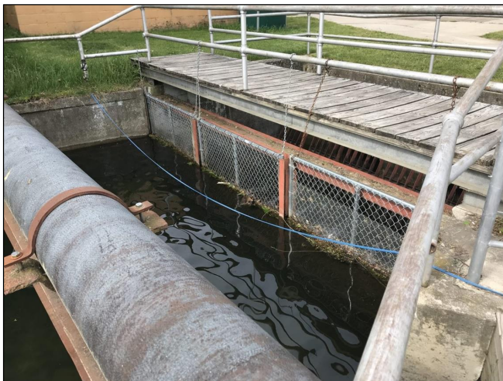
Photograph 18 – Upstream face of auxiliary spillway viewed from right wingwall.
