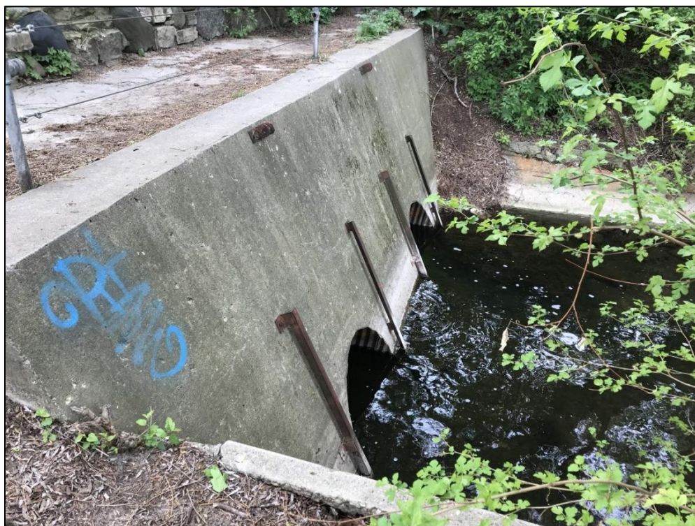
Photograph 54 – Auxiliary spillway outlet viewed from right wingwall.
