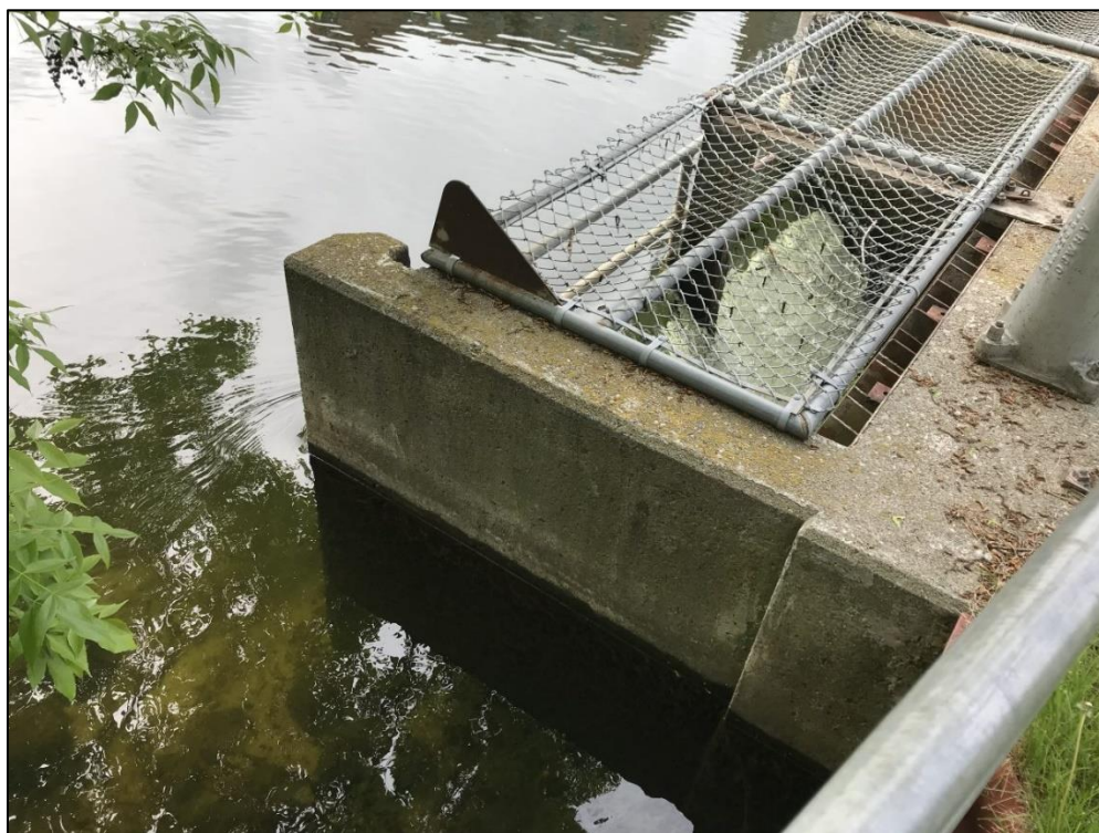
Photograph 31 – Right wingwall of primary spillway intake.
