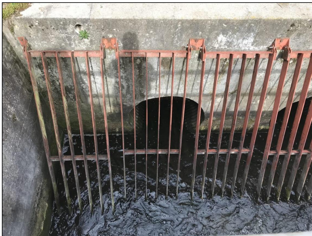
Photograph 7 – Left auxiliary spillway culvert inlet.
