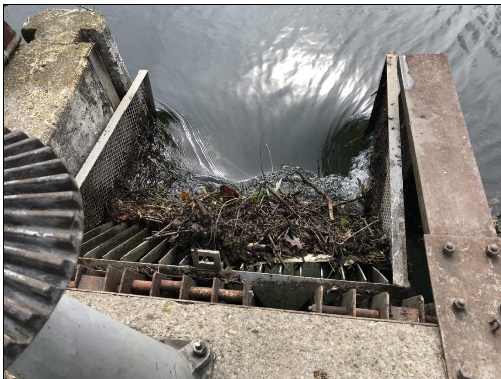
Photograph 28 – Right center bay of primary spillway intake.
