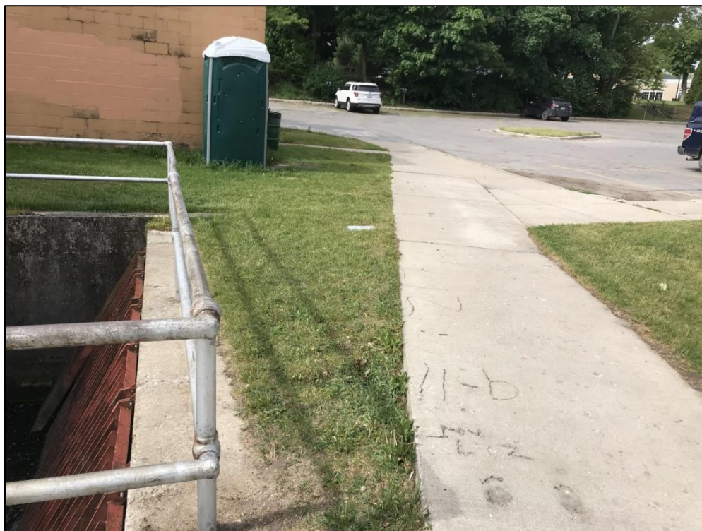
Photograph 9 – Crest of embankment over auxiliary spillway.
