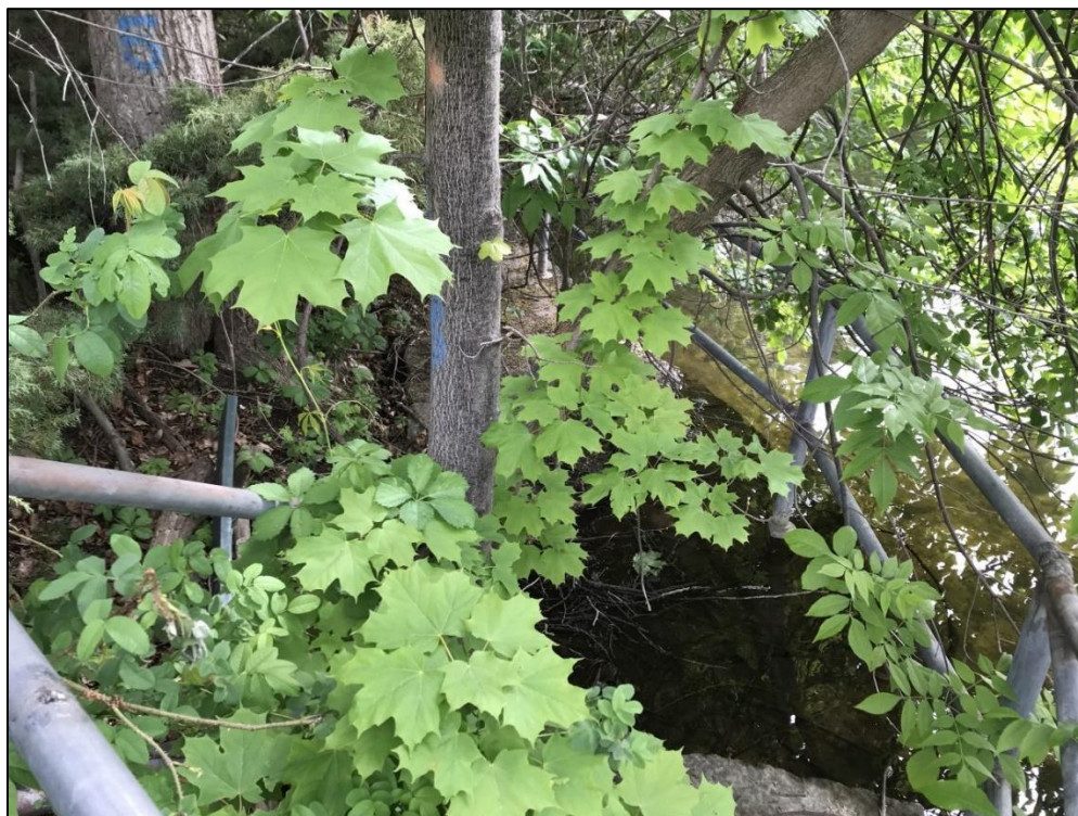
Photograph 32 – Looking at upstream right bank from right abutment.
