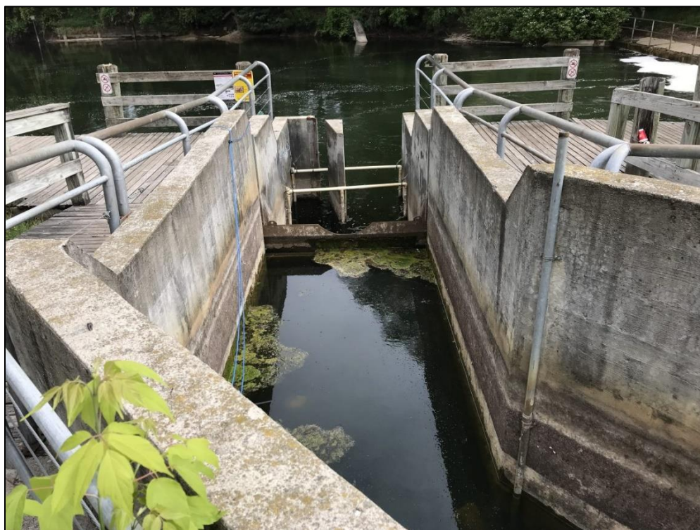
Photograph 52 – Looking downstream at fish ladder entrance.
