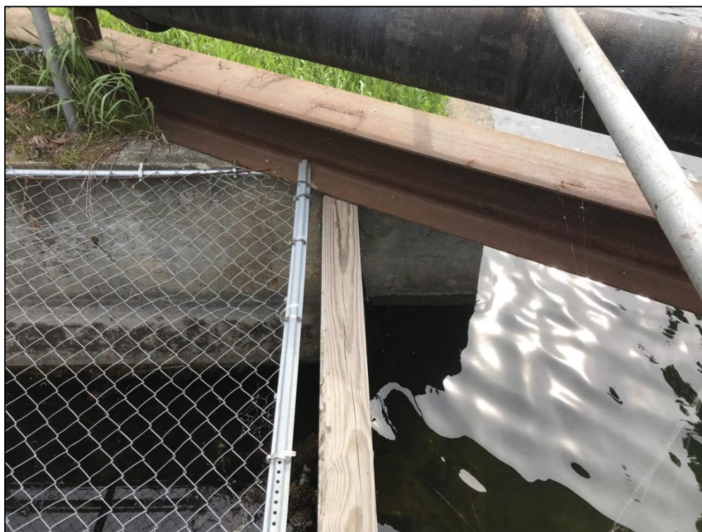
Photograph 10 – Stoplogs closing upstream end of fish ladder.
