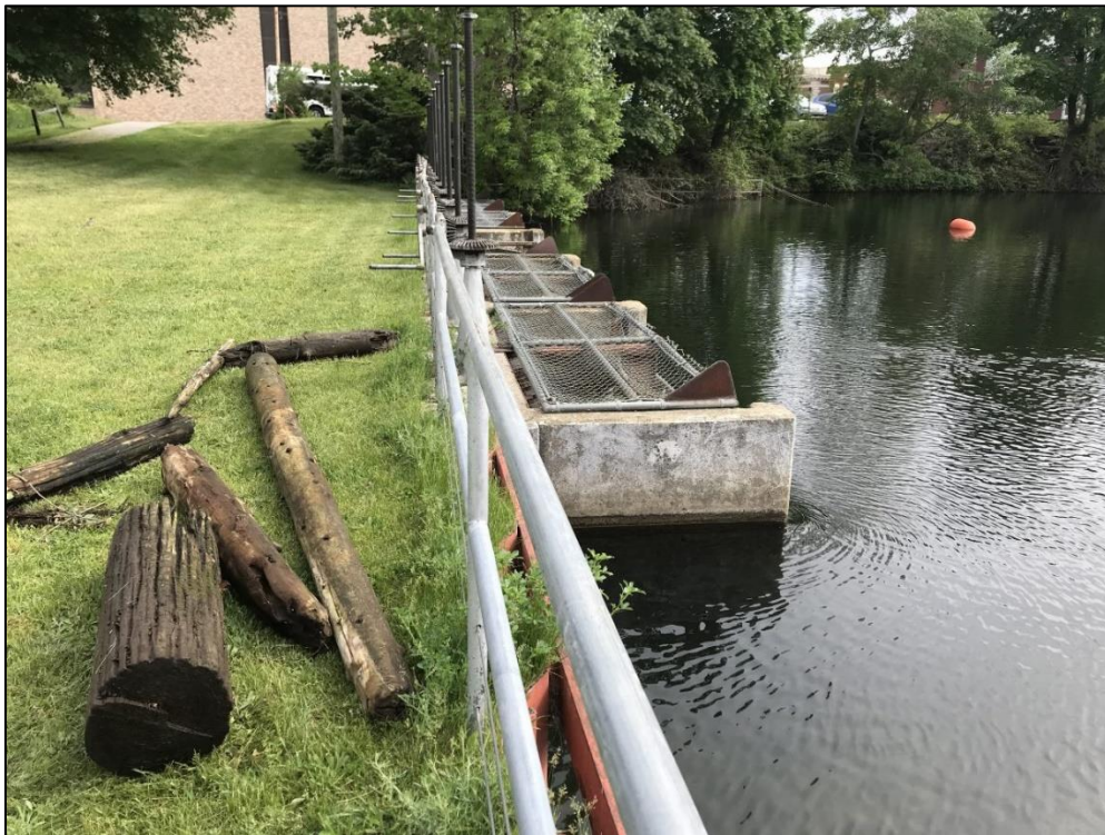
Photograph 22 – Upstream face of embankment and primary spillway. Note recently removed debris.
