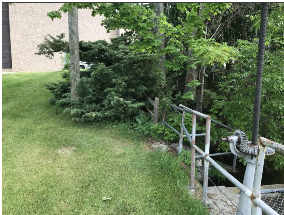
Photograph 29 – Upstream right abutment. Note trees and vegetation.
