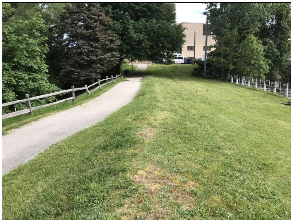
Photograph 16 – Crest of embankment viewed from fish ladder.
