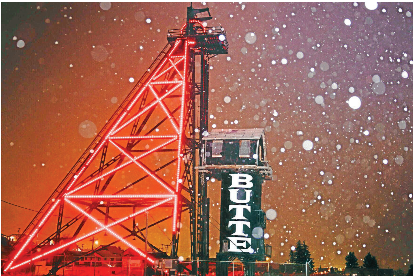
The Travona's newly replaced lights shine brightly into a blustery, snowy Tuesday night on May 7, 2024 in Butte.
