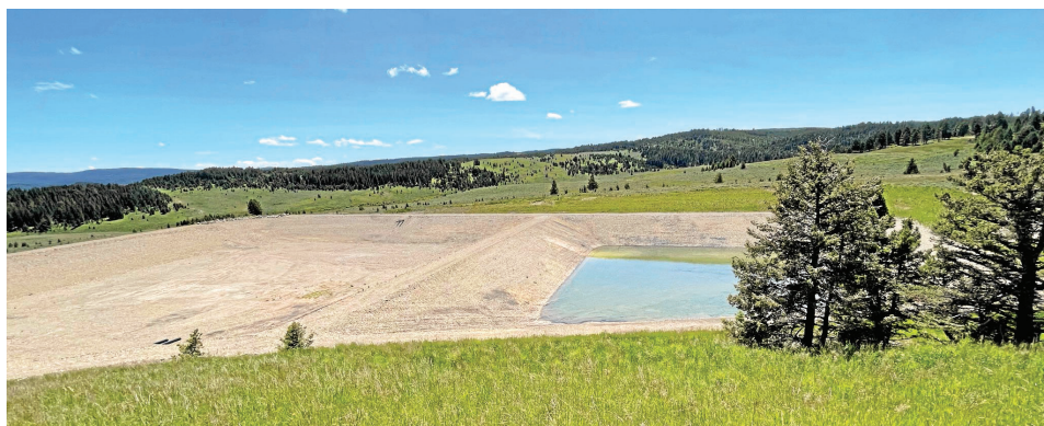
Two of the ponds which were built as part of the phase one construction work at the Black Butte Copper Project.
