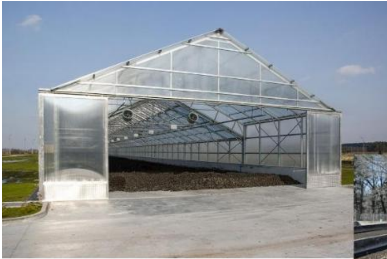
Solar Sewage Sludge Drying Facility
