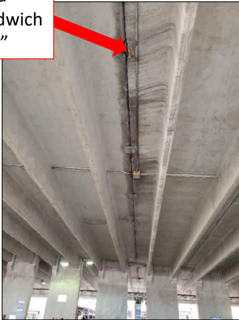
"Sandwich Plate" Joint
