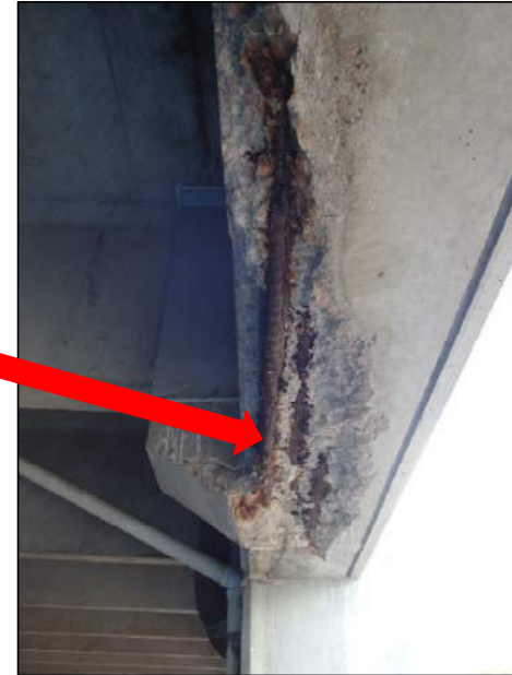
Damaged Spandrel on North Wall of Ramp
