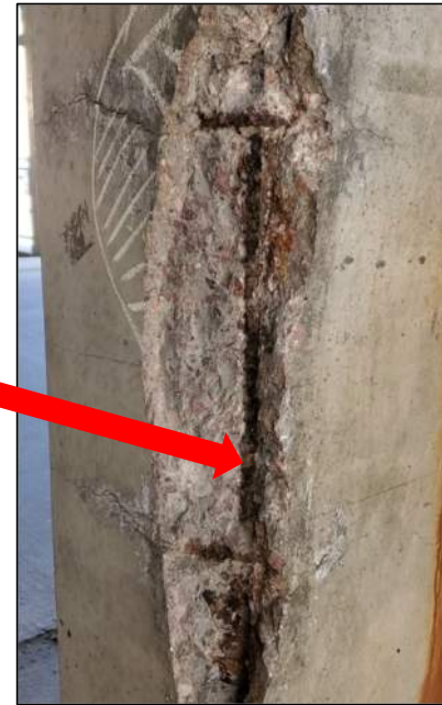
Damaged Column at East Stairs
