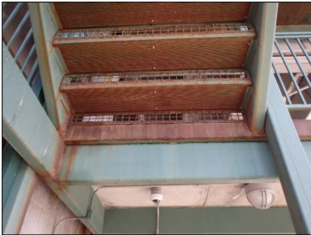
Rusted Stair Pans Typical Throughout
