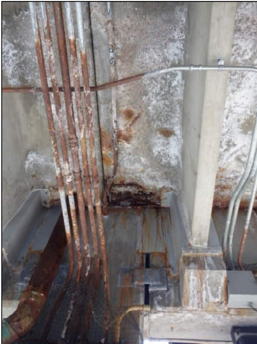
Corroded Electrical Conduit
