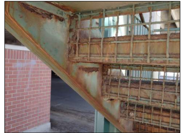
Corroded Stringers and Stair Pans
