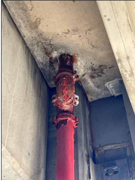
Rusting at Bend in Drain Pipe
