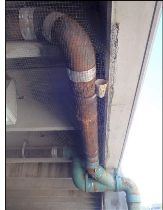
Completely Rusted Downspout
