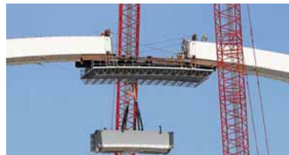
MAY 6, 2020: Standing 236 feet above the Mississippi River, crews await the 112.5-ton keystone piece.
