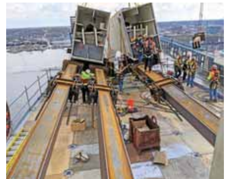
APRIL 23, 2020: Workers install struts to help with the keystone installation for the westbound arch supports.
