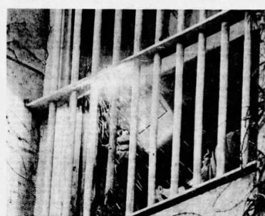
A wider repairs jail bars at the Scott County Jail Thursday after three juveniles saved their way free, escaped through, and apparently jumped about 15 feet to the ground. One of the youths later turned himself in. (Times photo by Bruce Hennessey)
