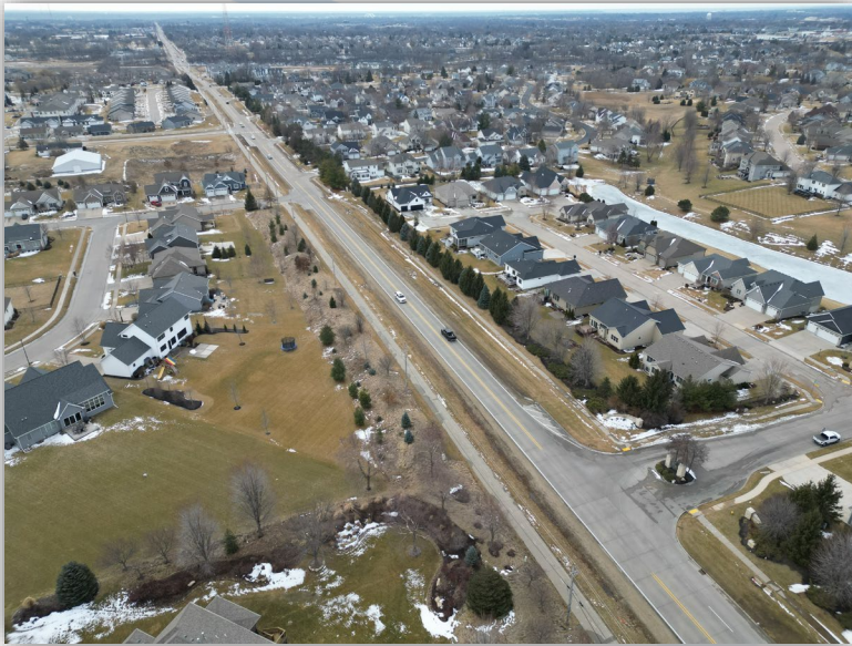
Construction Phase 2: Devils Glen Road Widening Project (53 rd Street to Crow Lake Drive)
