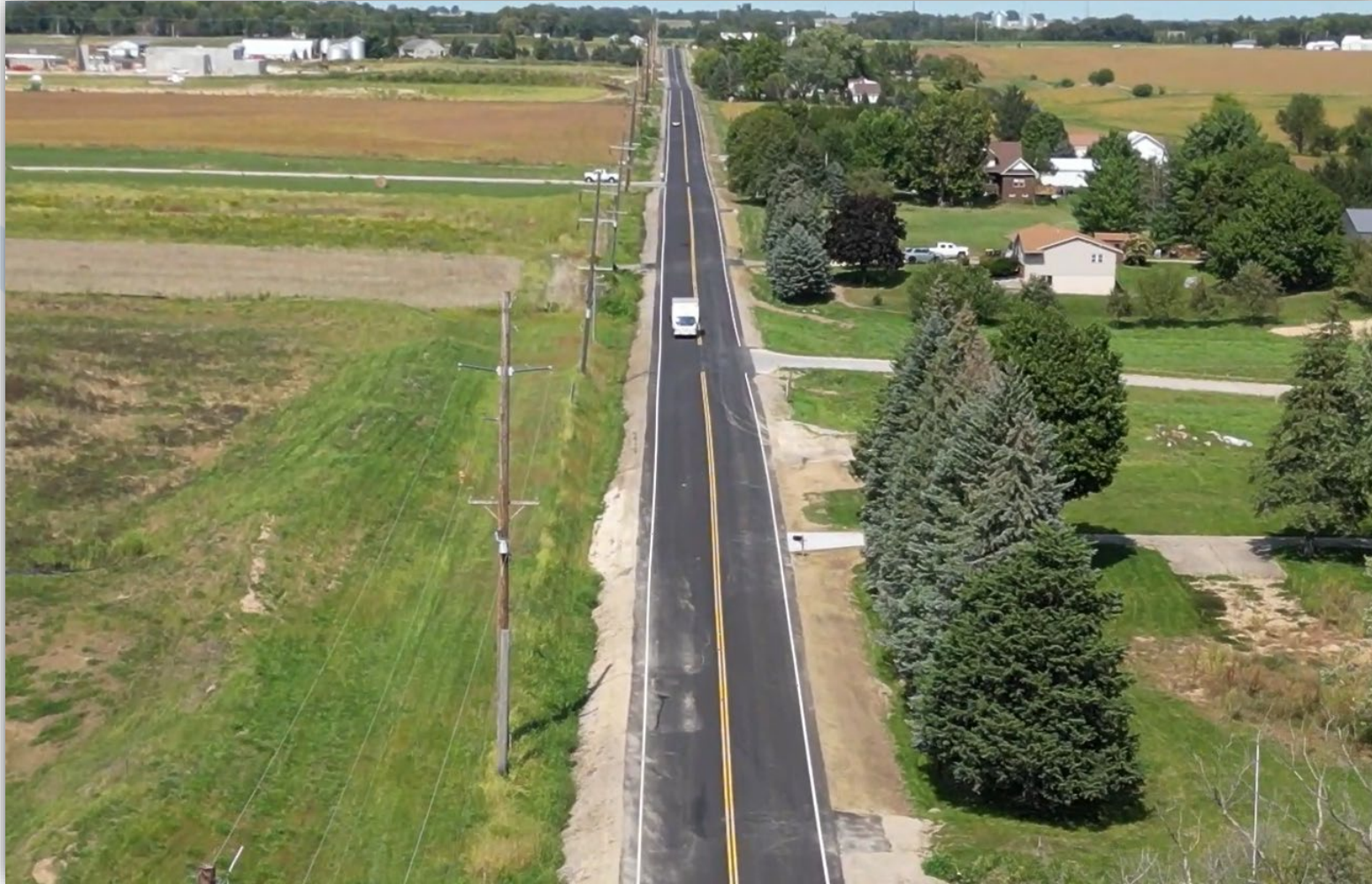
Criswell Street Rehabilitation Project 2024
