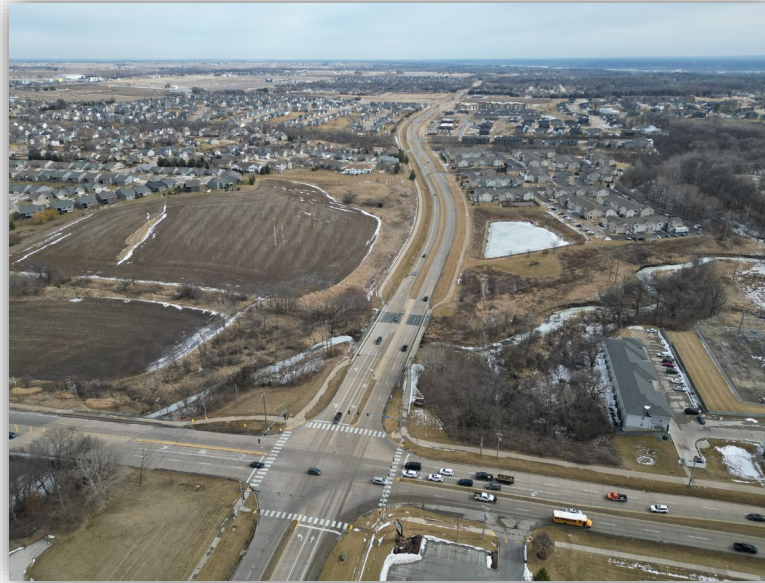
Construction Phase 1: 53 rd Avenue Widening Project (Devils Glen Road to Middle Road)
