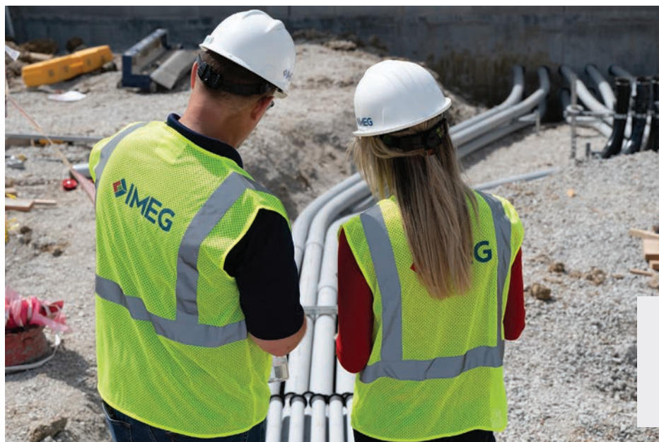
Matt Bowman , senior mechanical designer 2, and Kaylee Golden , electrical design technician, review site work. IMEG
