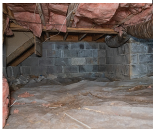
Crawl Space Encapsulation
