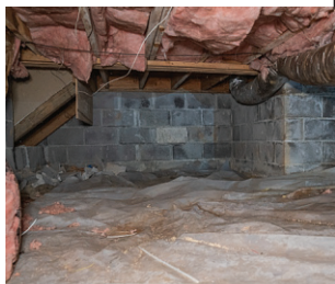
Crawl Space Encapsulation
