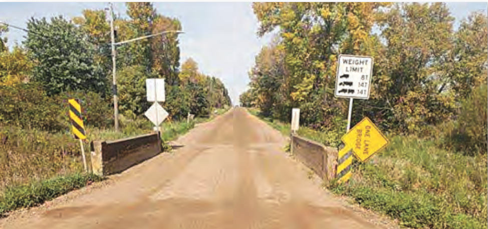
The Forest Road bridge, which is over 100 years old, is located just north of 175th Street, just west of Highway 61 and the Hardwood Creek Regional Trail.
