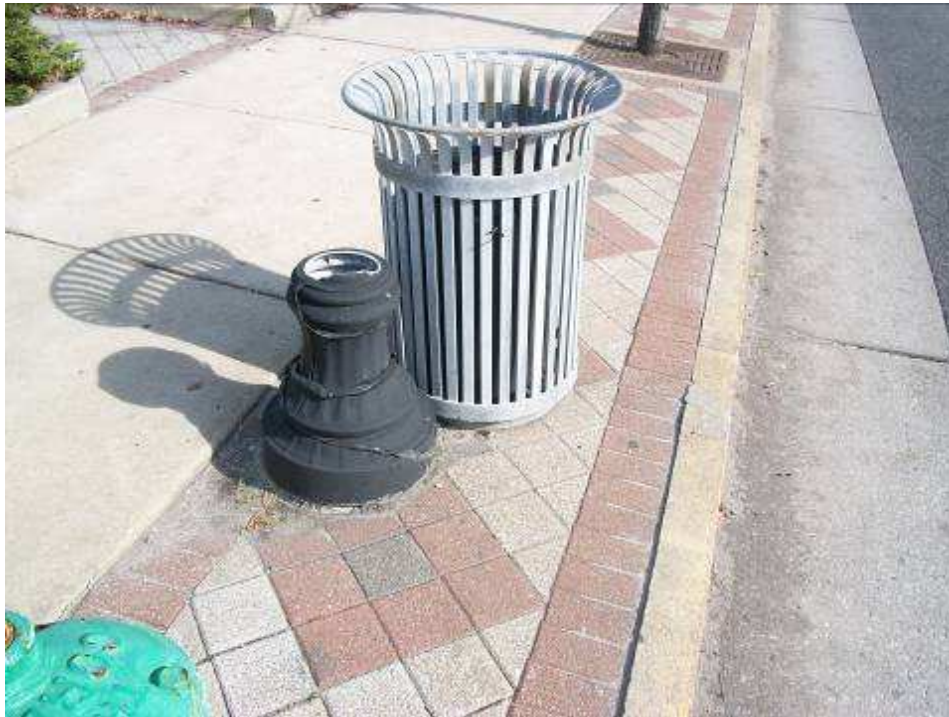
Photograph 11: Broken lighting fixture.
