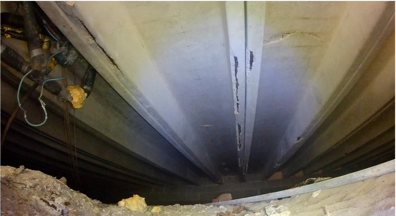
Corrosion of reinforcement and concrete spalling in some of first floor beams (crawlspace 1)
