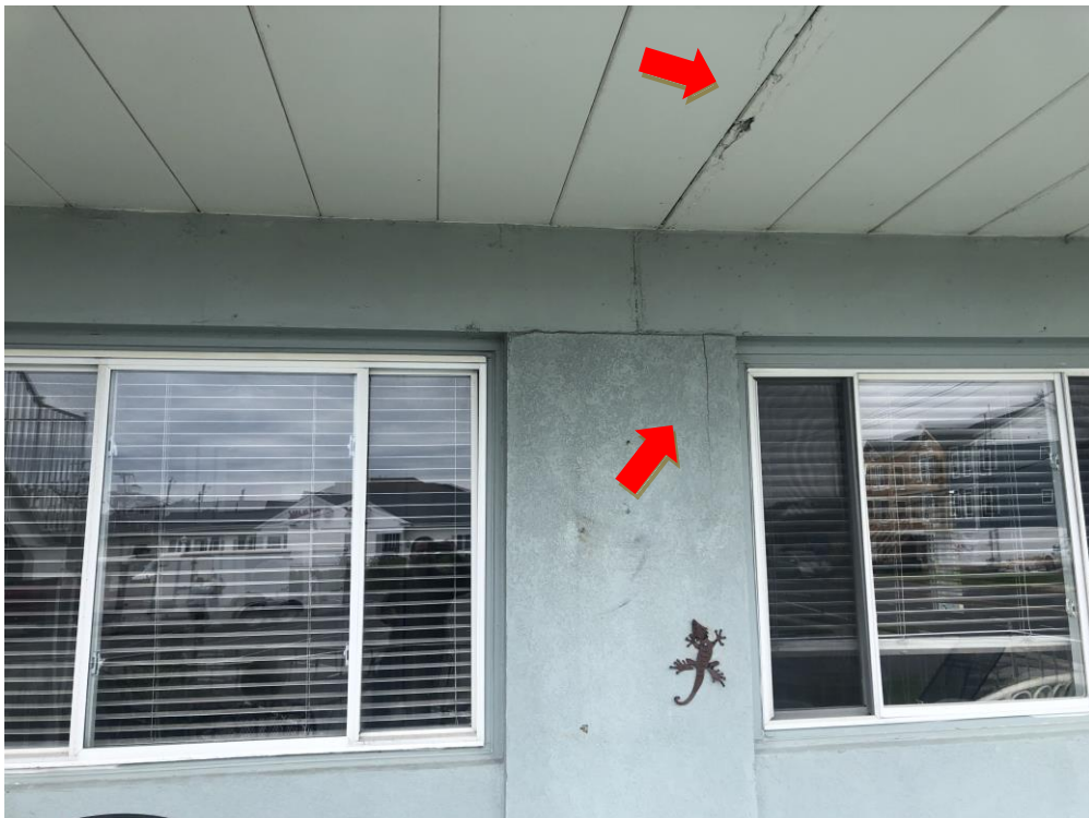
Northeastern side (Units 14 and 30) Note limited wall cracks
