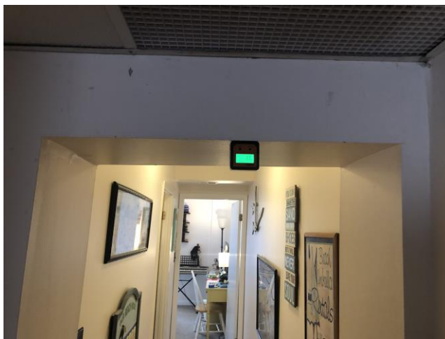
(Units 19+32 – interior) No visible cracks
