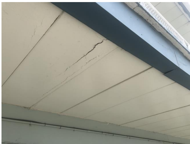
2 nd Floor walkways Note cracks with need of repairs or restoration
