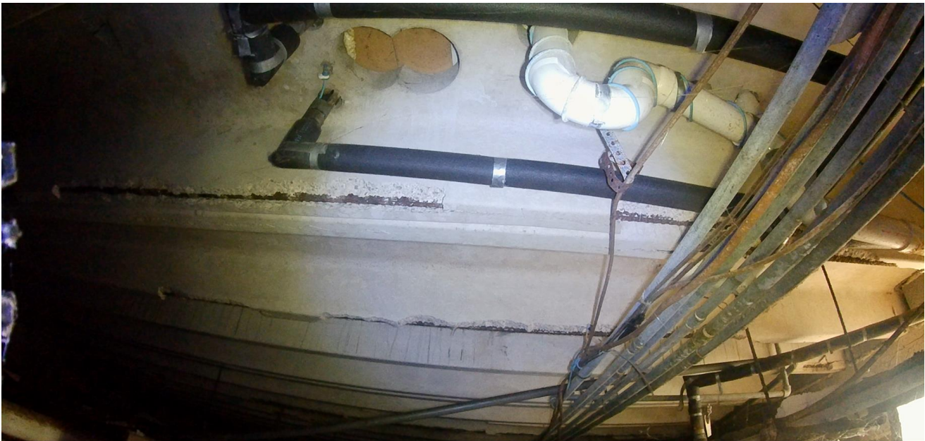
Corrosion of reinforcement and concrete spalling in a few of first floor beams. Most are likely caused by chipping activities (crawlspace 2)
