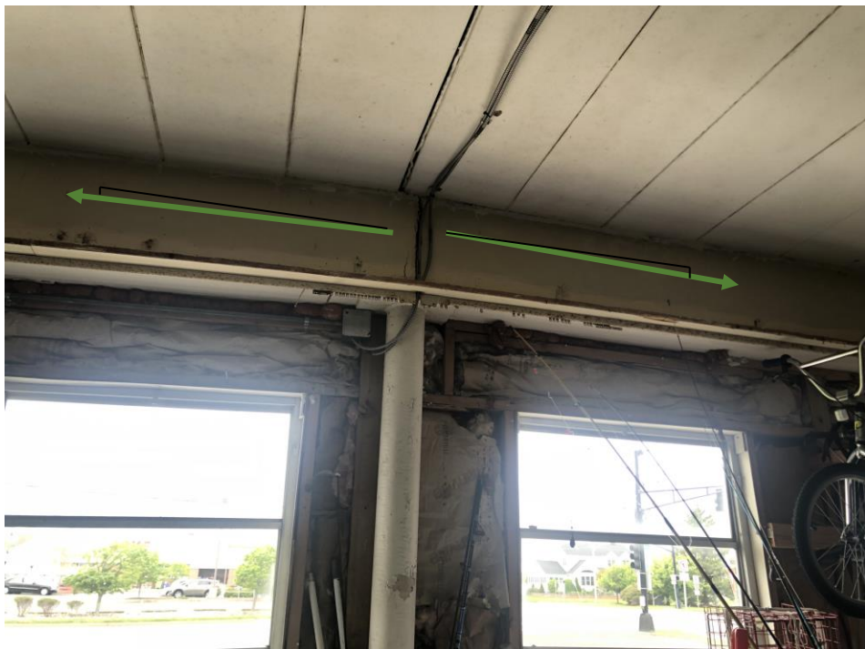
(Storage Room) Note the lintels pitched (by design) to facilitate roof drainage
