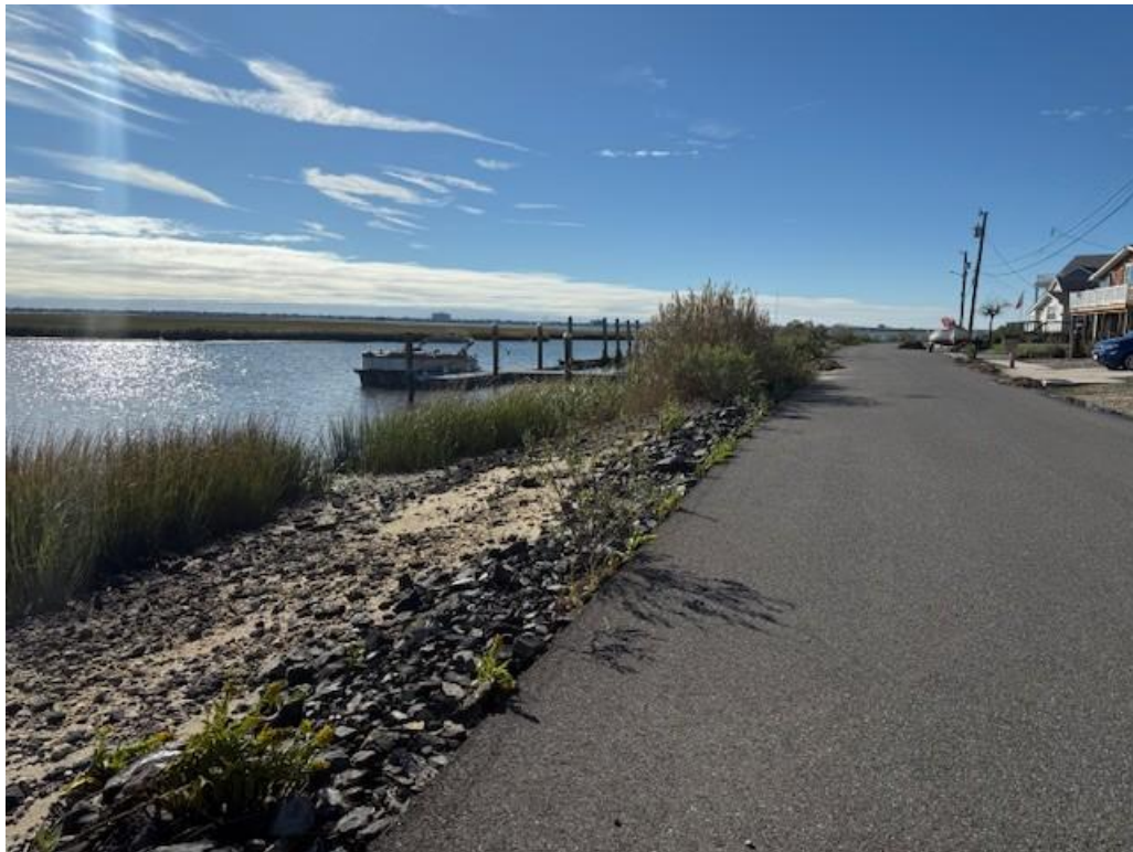
Bulkhead along O'Byrne Drive
