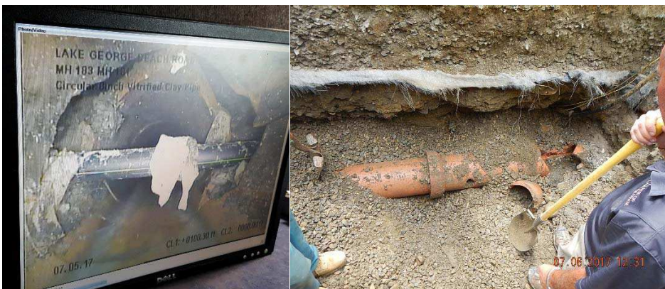
Broken sewer line and actual photo from camera inspection
