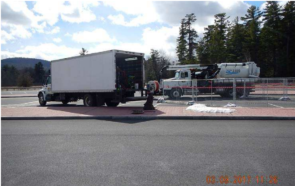
Video camera inspection truck
