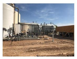
Ion exchange (IX) technology is widely recognized as a proven and cost-effective method of removing nitrates from water. At the Johnson Utilities Main Yard, the new IX system has now been up and running for several weeks. Installing equipment of this size and level of complexity normally entails some commissioning adjustments. We've largely worked through these issues and the system is meeting our expectations for treating groundwater in the region to bring it into water quality compliance.
