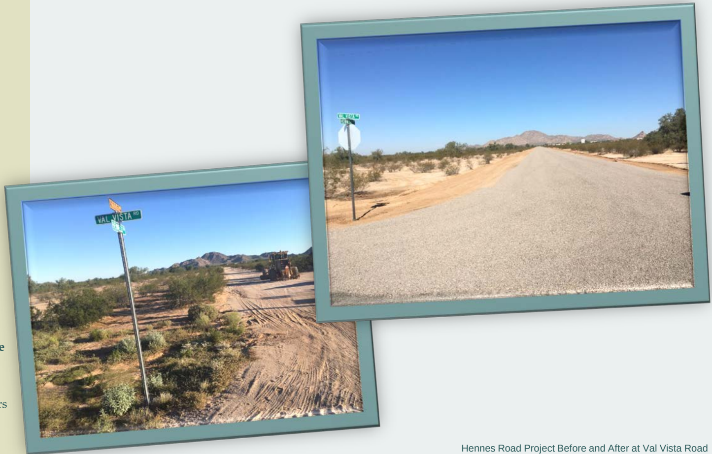
Hennes Road Project Before and After at Val Vista Road
