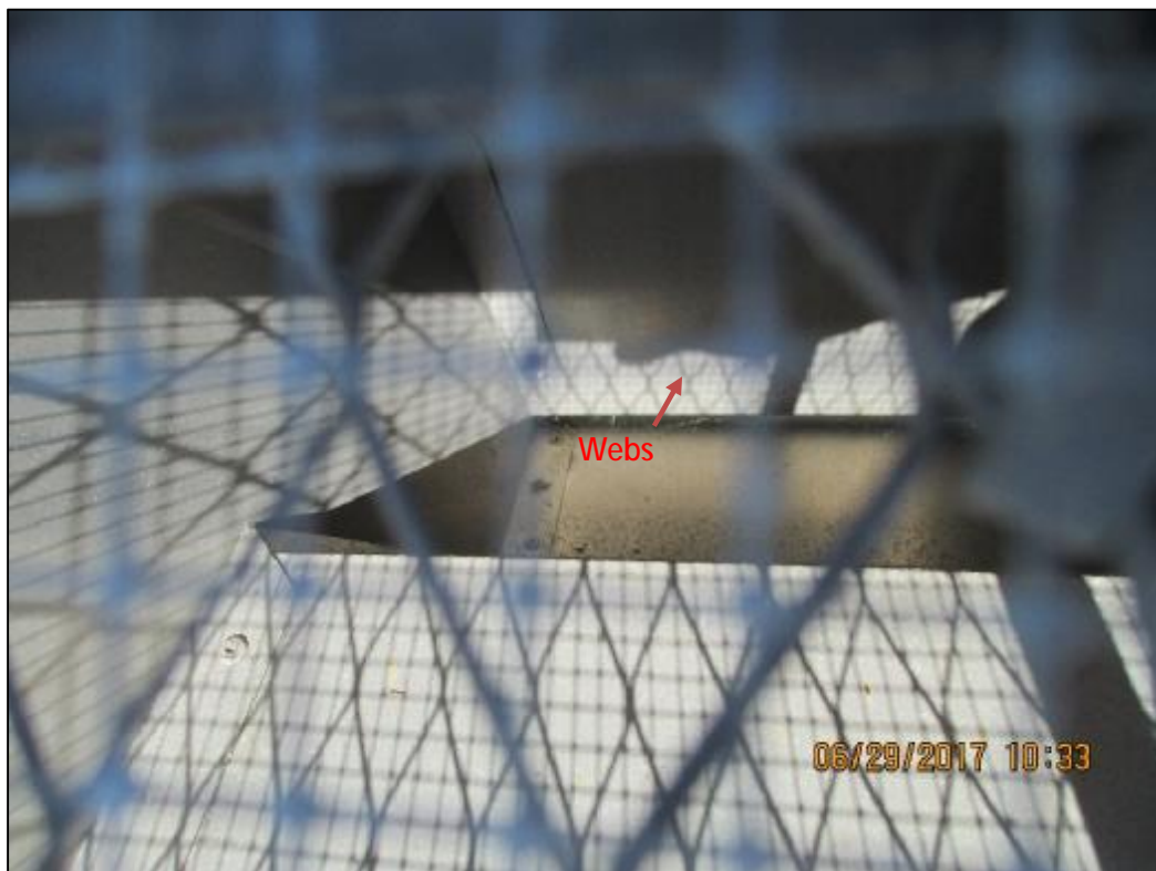
Photograph 4: Reservoir 51771's vent mesh is too wide, as evidenced by a spider and webs living within the vent.
