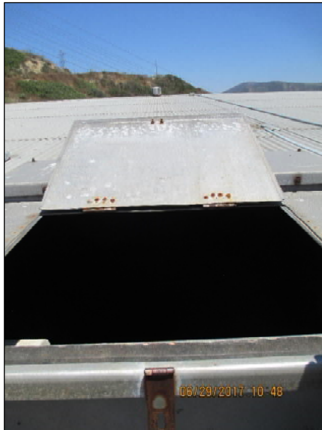
Photograph 8: Reservoir 51772's hatch was flush with the roof.
