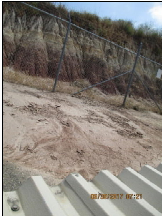
Photograph 19: A hill near Reservoir 63210 was eroding and depositing loads of dirt immediately adjacent to the reservoir.
