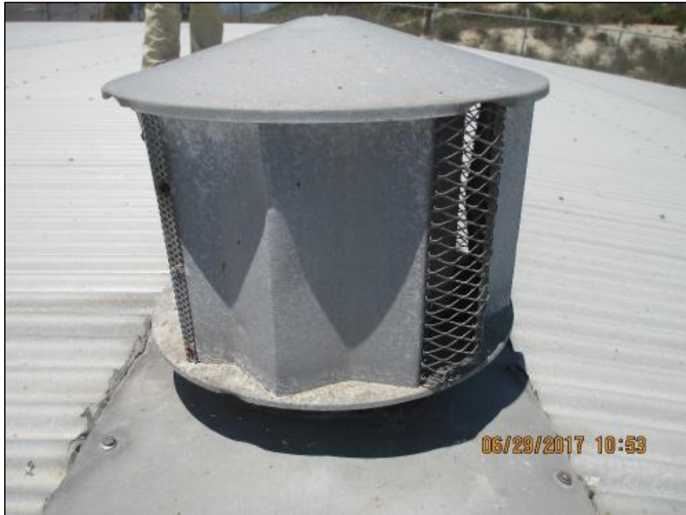
Photograph 9: Reservoir 51772's vent did not have a 24-mesh screen and protection from rain and airborne contaminants.
