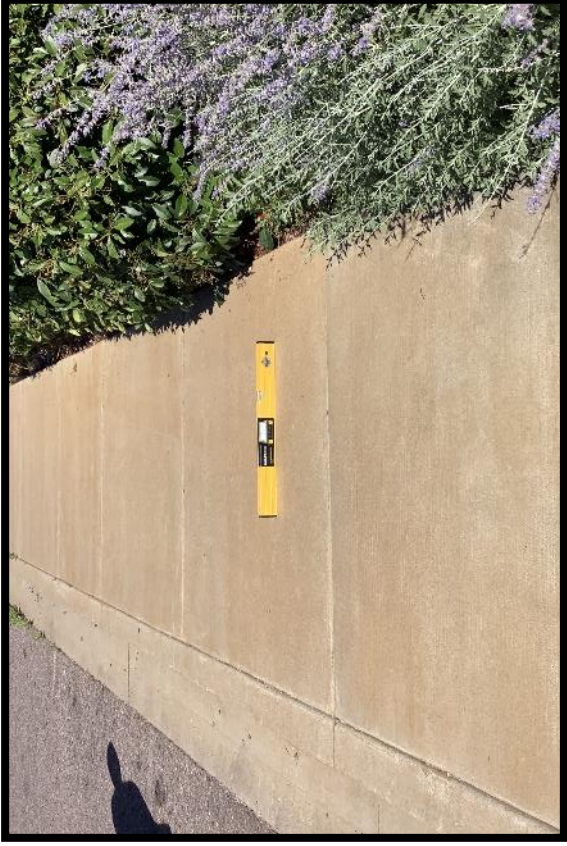
3.5% CROSS SLOPE ALONG SIDEWALK
