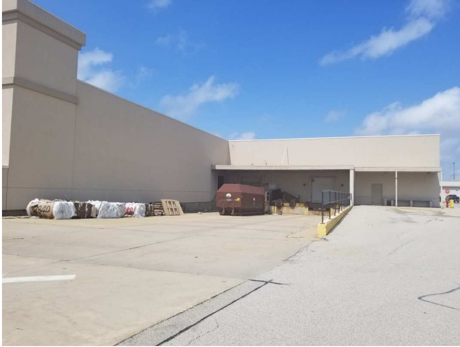
Sears Loading Dock
