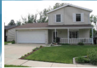
14 Carraway, BL • $129,900 Great spacious 2 story in the Lakewood area. Formal living room, dining and family room spaces. Enclosed 3 seasons porch off the back, fully fenced backyard with lush landscaping and patio. Quiet cul de sac location, 2 car garage. A great move in ready home!
