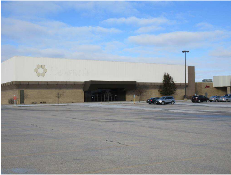
Former Bergner's Anchor – East Side
