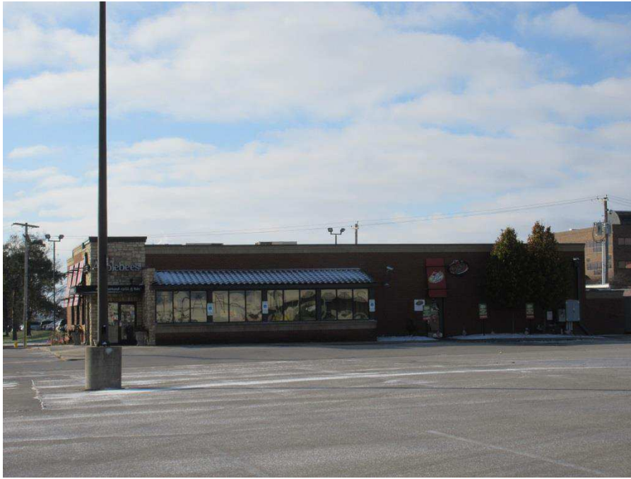
Applebee's Outparcel – Southeast Corner
