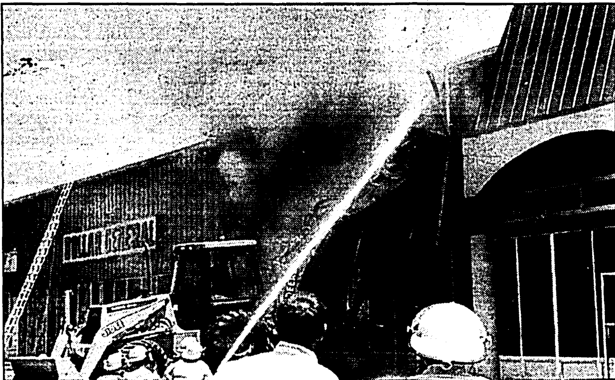
Getting at the fire Ron Creagan, city street superintendent and firefighter, operated a backhoe to tear apart the front wall of the mall building on Wednesday afternoon. Firefighters had to remove parts of the wall to extinguish flames burning between the ceiling and the roof of the building.
