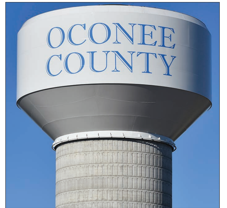
The new water tower off U.S. 441 near Watkinsville is 141 feet tall and holds 750,000 gallons of water. [Photo by Michael Prochaska]
