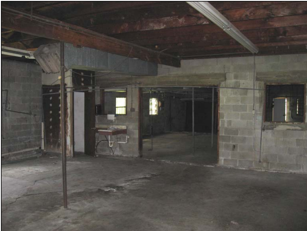
8. Former Fallo's Cleaners interior.
