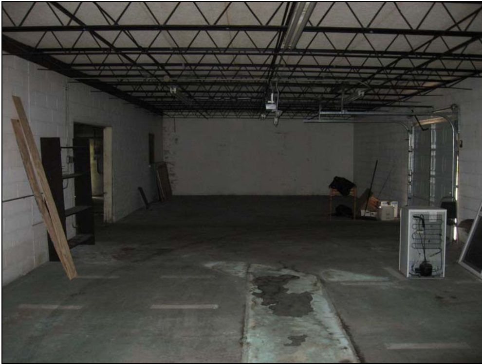
9. Former Fallo's Cleaners interior.
