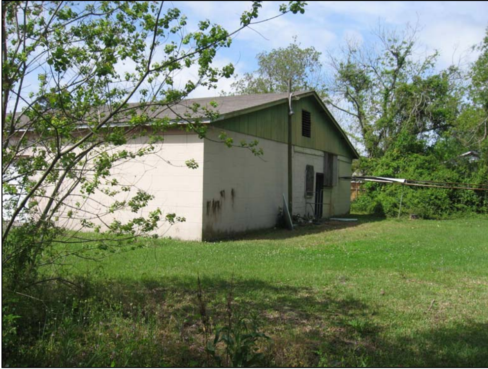
5. Rear of former Fallo's Cleaners.
