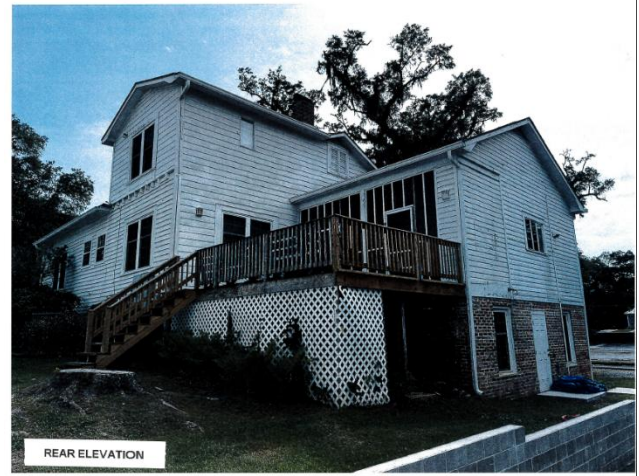
Figure 2,3,4,5. Existing Deck and Screened Porch
