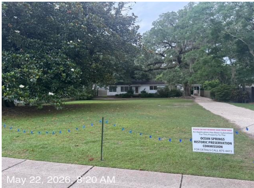
Figure 1: Historic Planning Commission Signage
