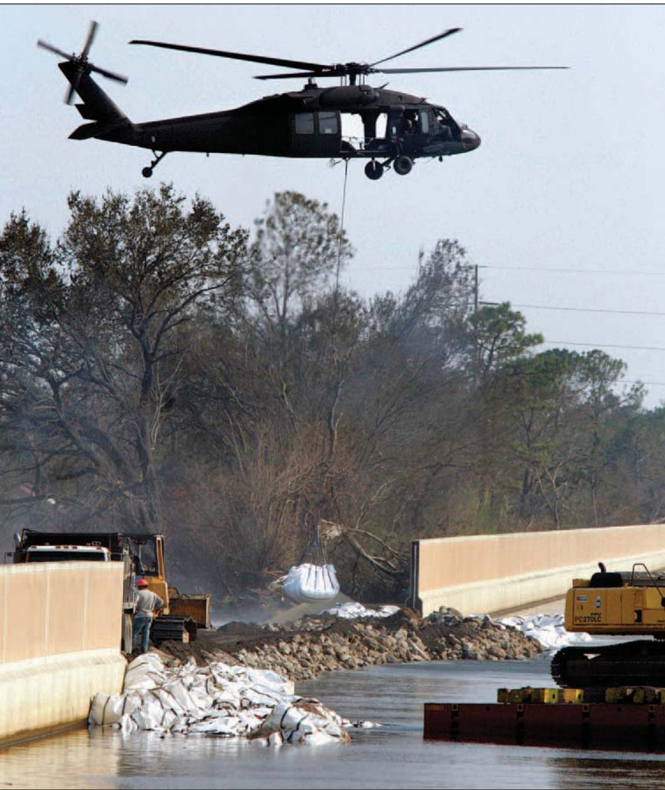
Plugging a breached floodwall, New Orleans
