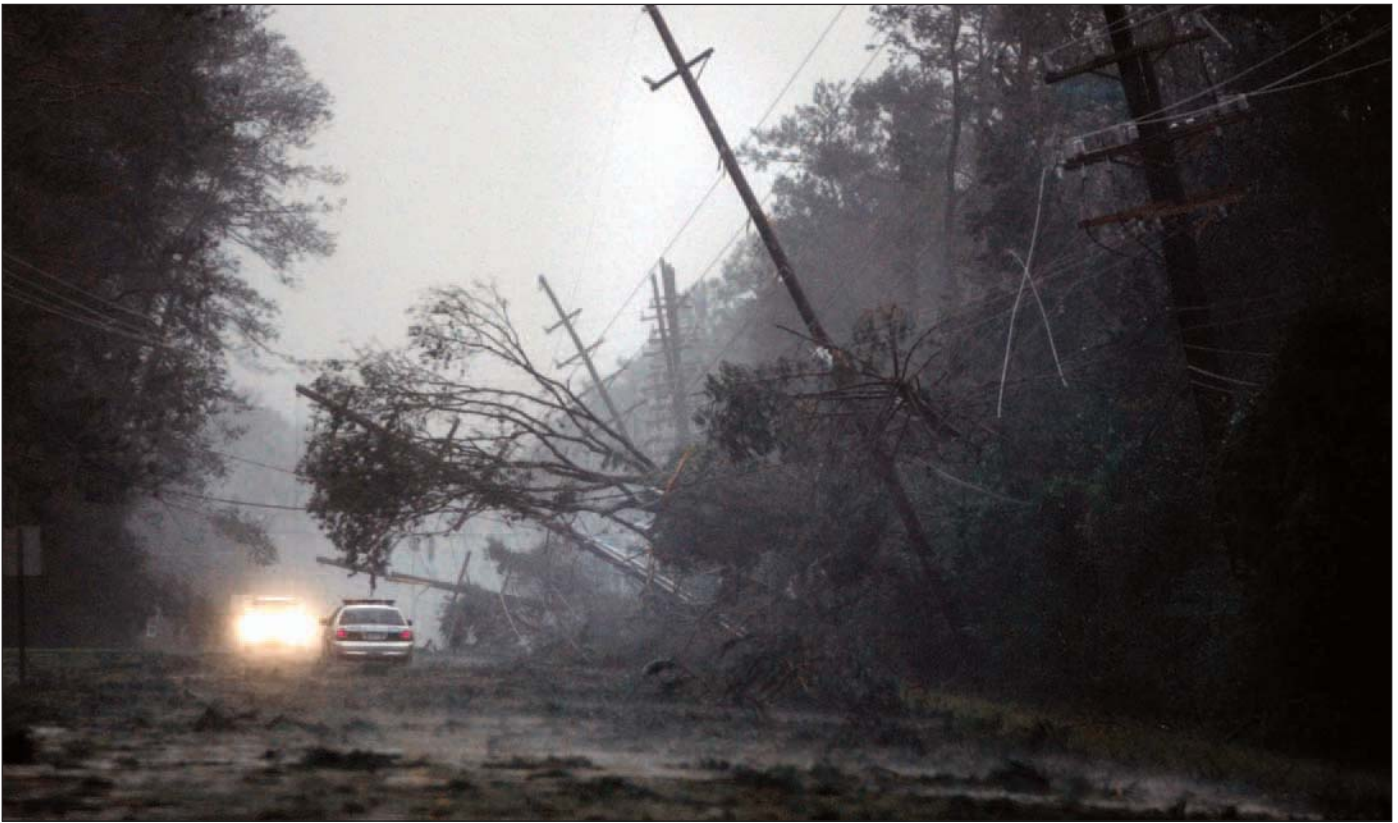
Broken utility poles, Mandeville, LA
