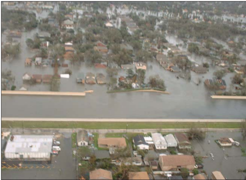
Breached floodwall, New Orleans Marty Bahamonde photo
