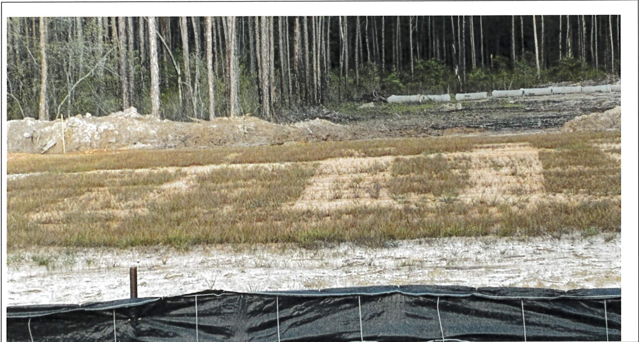
Photo 7: Looking east from Gibson Road, behind proposed lots 40-52; there is no erosion control between the current grading and forested wetlands/conservation easement
