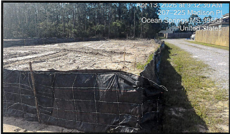
Silt fence will be removed from drainage conveyance and vegetation will be planted to restore impacted area.
