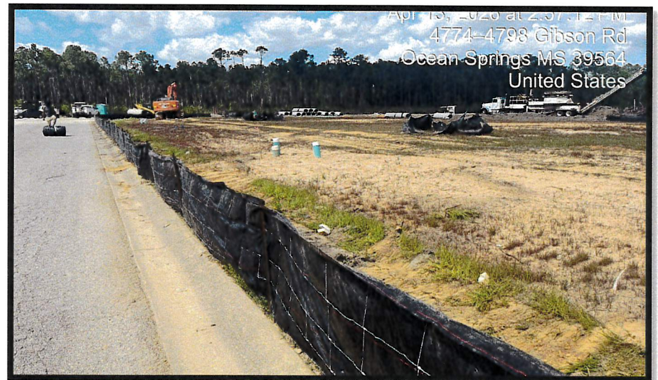
View of repaired silt fence
