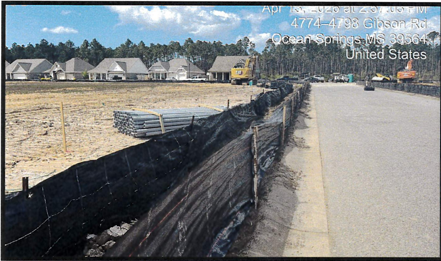
View of double row silt fence
