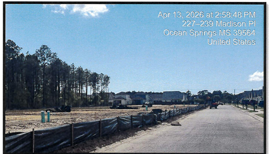
View of repaired silt fence
