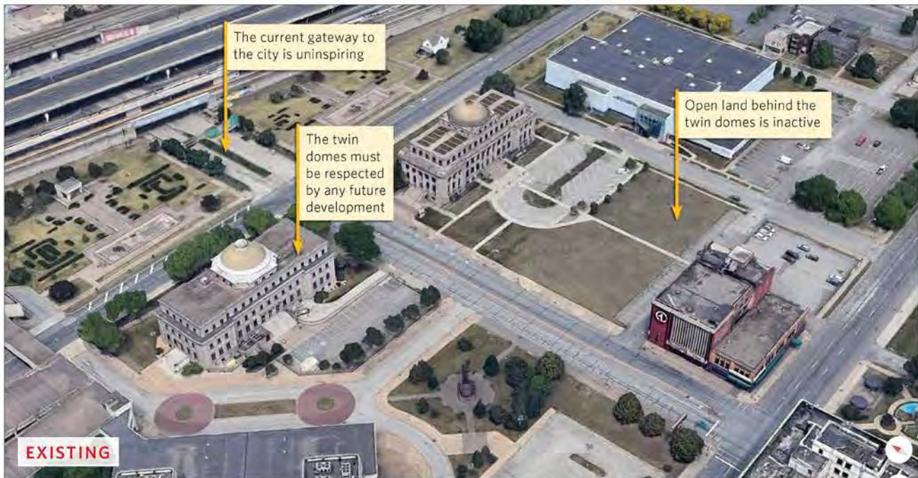
FIGURE 58: Aerial View of the Existing Site
