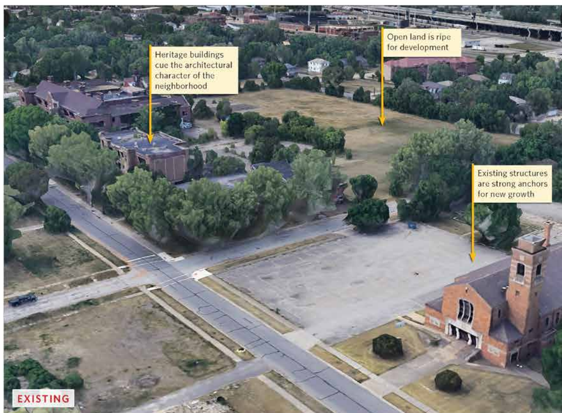
FIGURE 66: Aerial View of the Existing Site
