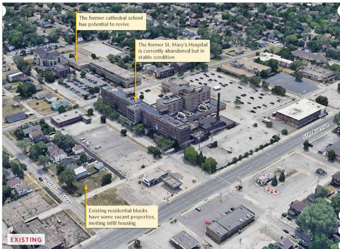
FIGURE 74: Aerial View of the Existing Site
