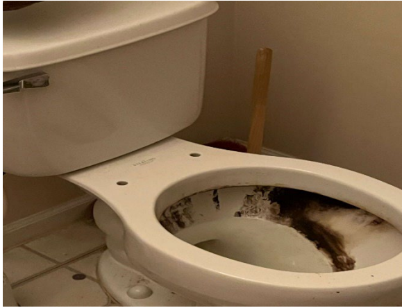
Photograph 3: Missing toilet seat and mold in toilet
