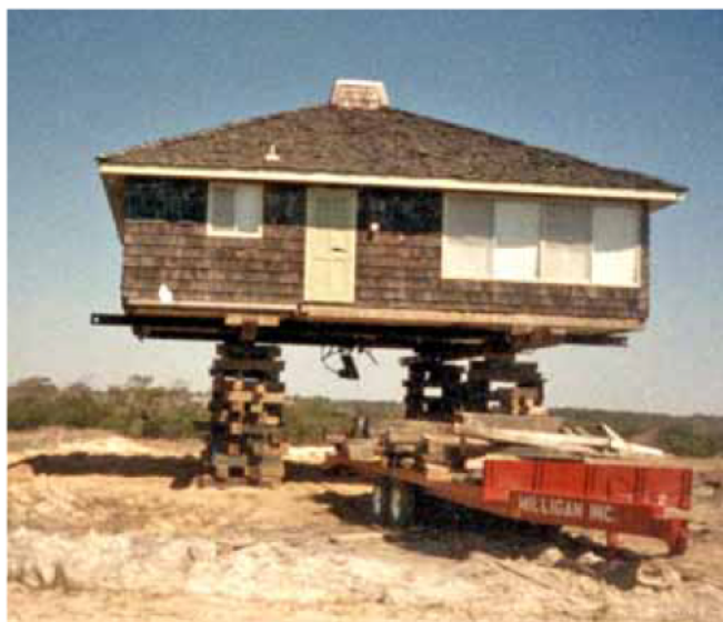
Cribbing up a building before moving.
