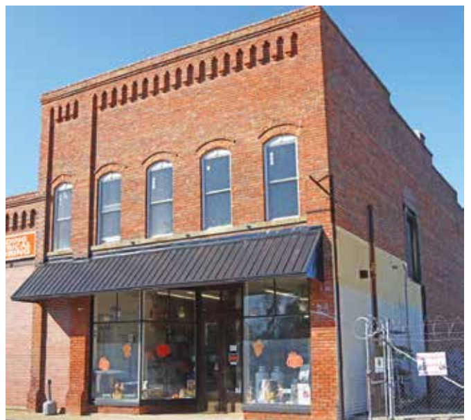
The McArthur Supply store was built in 1905 and was the first hardware store built in Chadbourn.
