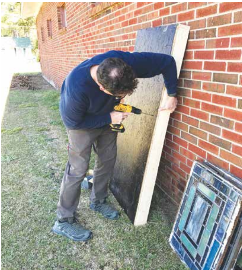
The sturdy frames were individually made for each window prior to their removal to storage pending installation in the new church building.
