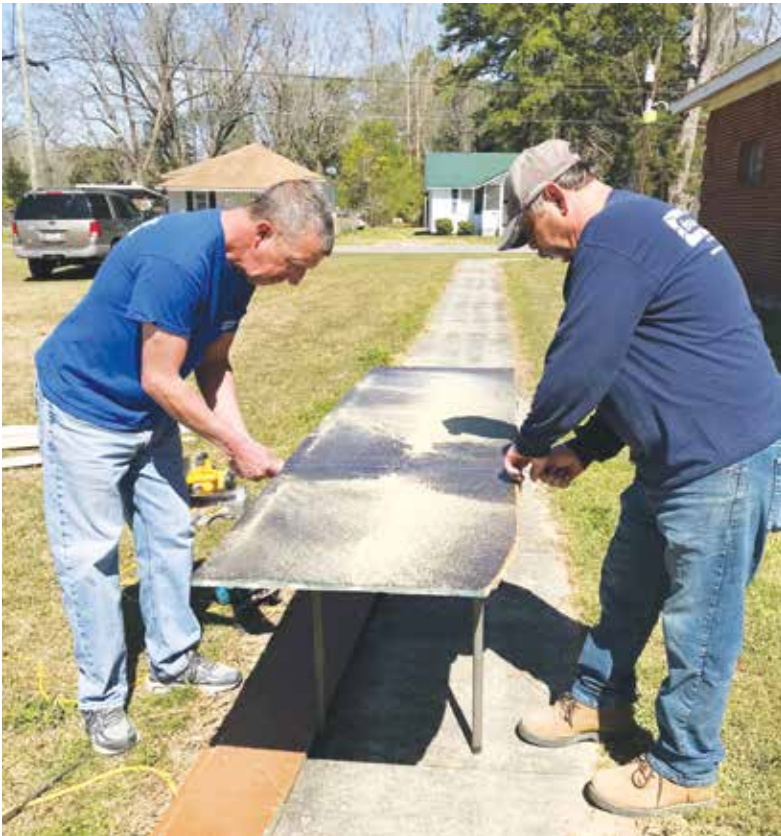
Employees of Strickland Stained Glass Associates prepare the frames to hold the windows removed from the church.
