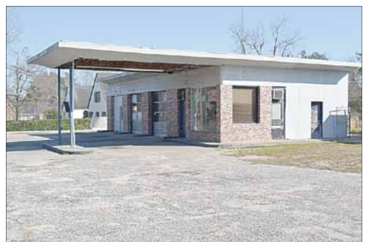
The old Grainger station is slated for demolition.
