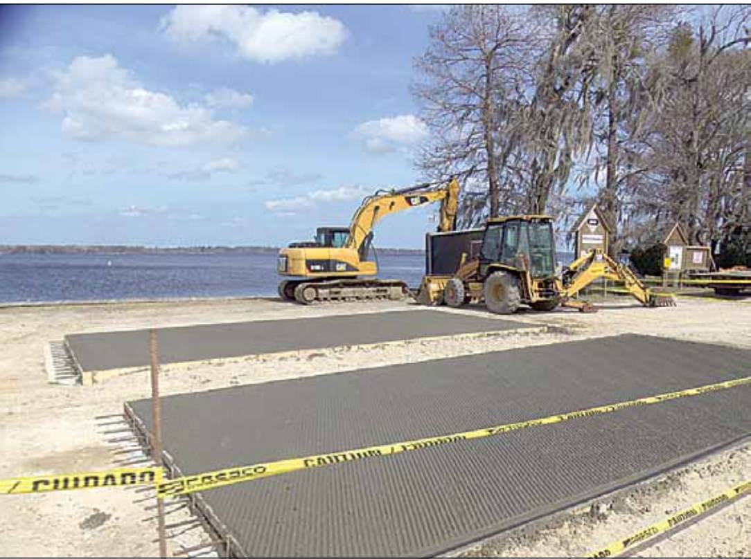
Construction has started on the Canal Cove Wildlife Resources Commission boating access area. Officials say the work will be completed by Memorial Day.
