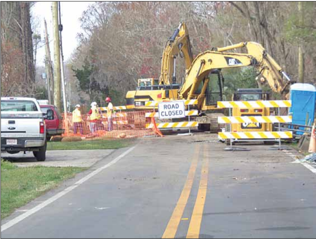
Work is continuing on the box culvert project that will replace the narrow bridge on Canal Cove Road at Lake Waccamaw.
