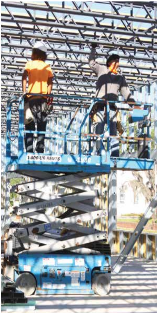
A pair of carpenters use a lift to reach the joists.
