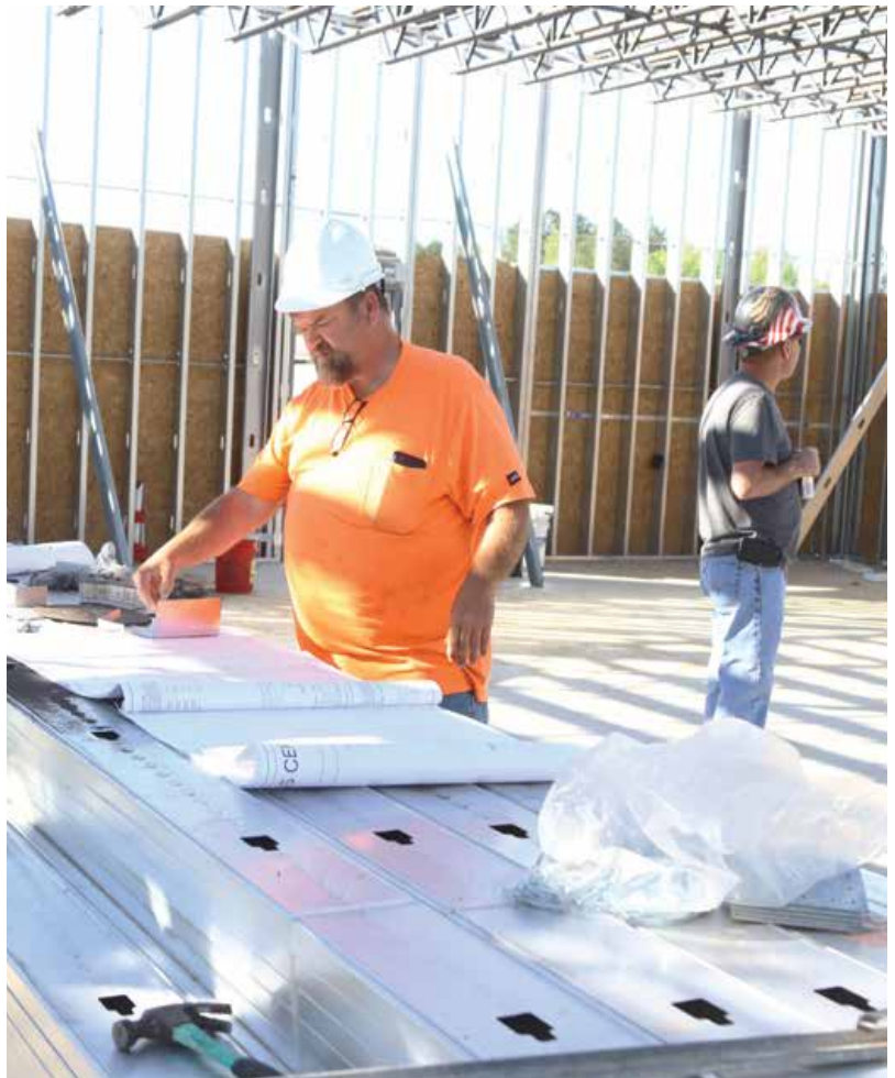
Carpenters install 2 by 4 nailers atop steel joists to support the upper floor.
