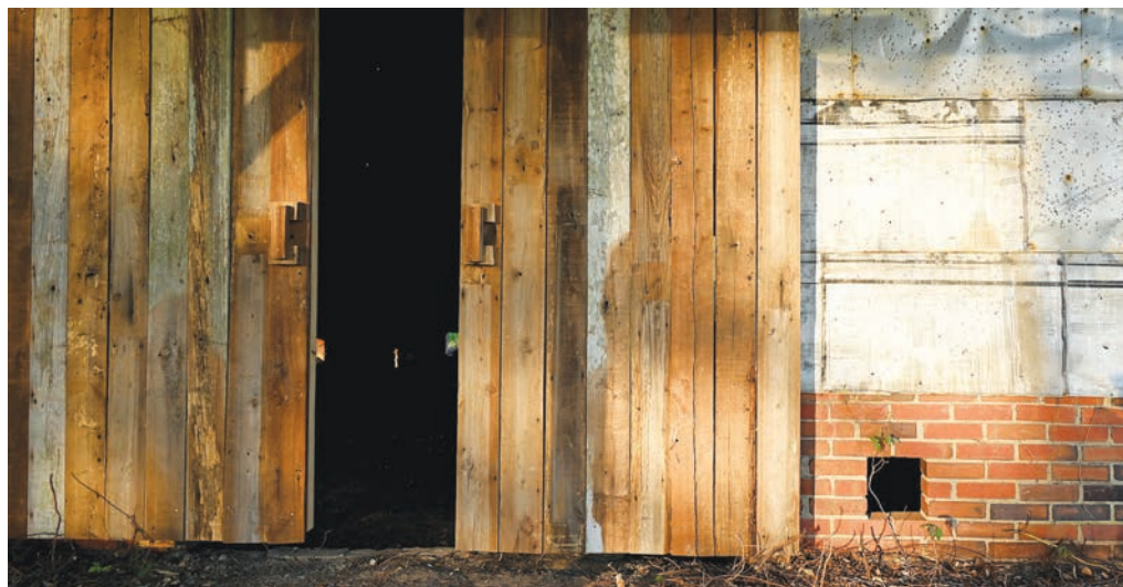
Lumber from an adjacent barn storm damaged beyond repair was repurposed to restore the last remaining tobacco barn on the High farm.
