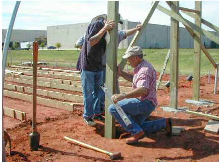
Use a string line attached to opposite ground posts to align end wall posts. A carpenter's level is needed when setting posts to ensure they are installed plumb.
