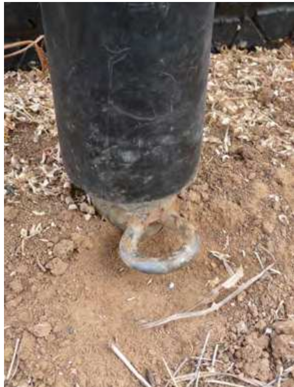
Eyebolt used to secure rope to ground posts
