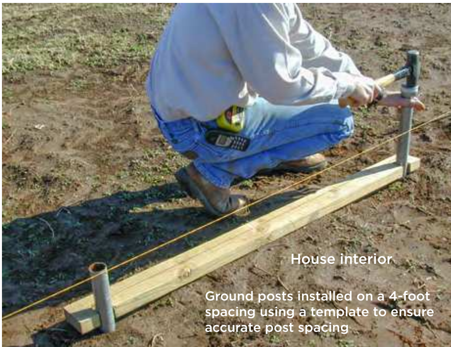
Accurate ground post installation minimizes complications that can arise during house construction.
