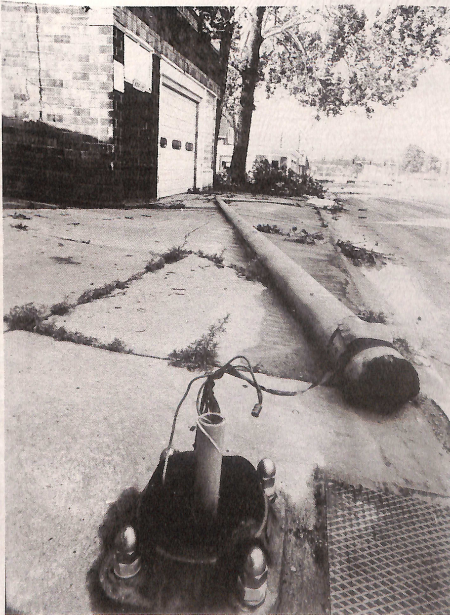
Straight-line winds clocked at nearly 100 mph at Eppley Airfield in Omaha caused extensive damage to the utilities in Council Bluffs. This power pole in the 500 block of East Broadway was sheared off at ground level by the winds. — Photo by Jon Leu.
